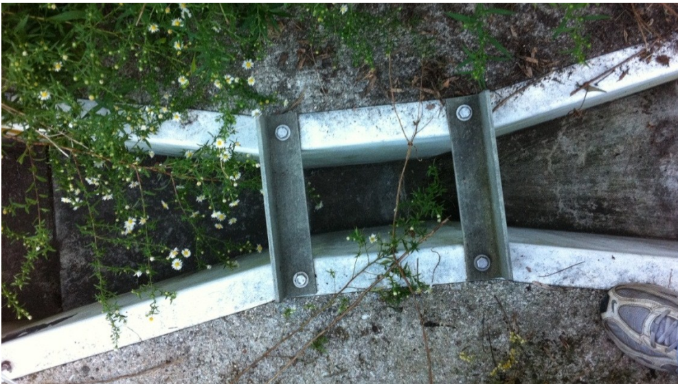
b. View over Parshall flume
