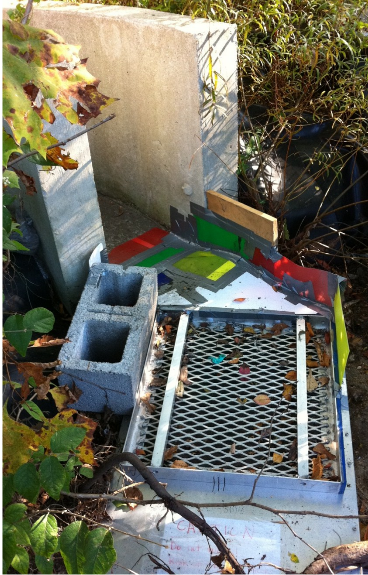
Figure 76. Prototype filter tub in place at end of runoff channel.
