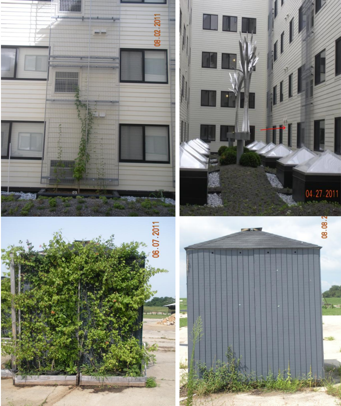
Figure 3. Green façades(left) and their associated control walls (right), from top to bottom: Eastern Village Cohousing apartments Takoma Park, MD; Avalon apartments parking garage Rockville, MD; National Wildlife Federation headquarters Reston, VA; Twinbrook Parkway parking garage Rockville, MD; RTKL office building Washinton, D.C.; Finnish Embassy Washington, D.C.; Montgomery College parking garage Takoma Park, MD; Alaire apartments parking garage Rockville, MD; Three Tree Flat apartments Washington, D.C.; experimental green façade structures Clarksville, MD.
