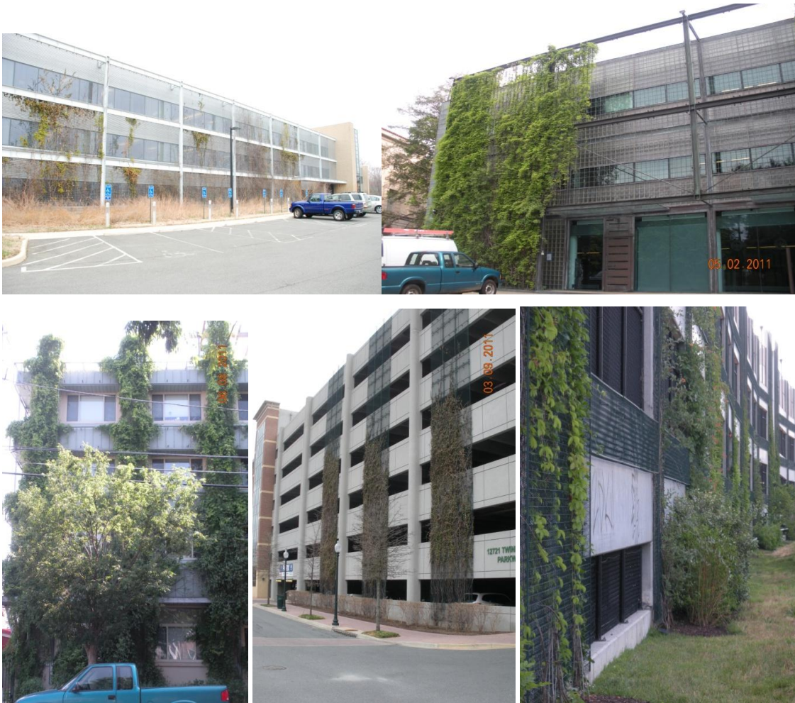
Figure 2. Installations varied in their configuration but all consisted of steel mesh panels fastened to steel frames, which were then mounted to a building façade. Some installations consisted of continuous panels (top images) while others consisted of panel broken up along the length of a building wall (bottom images).
