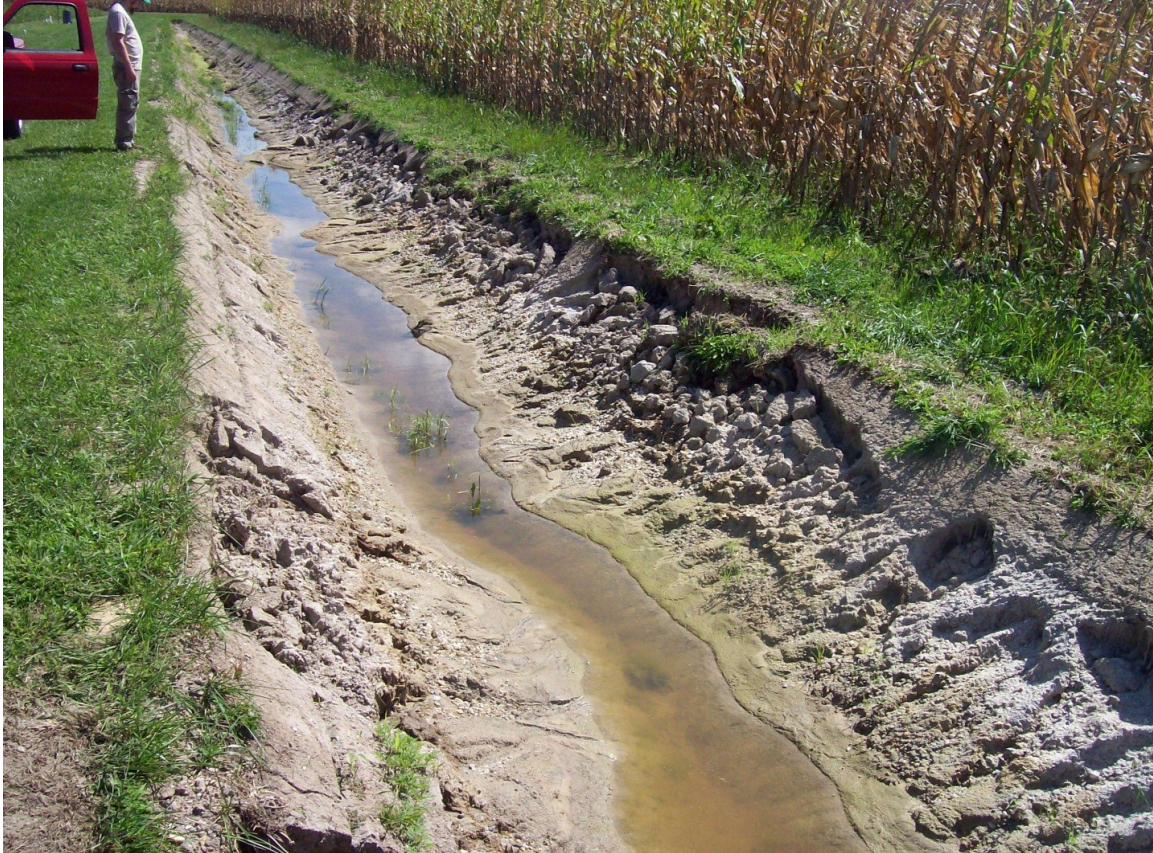
Illustration 3.4. Erosion of ditch banks several weeks after dredging. Note the slumped ditch sides, structureless materials occupying the channel, inclusions of former A horizon material with plants occasionally in the channel, and lack of vegetative growth on ditch banks.
