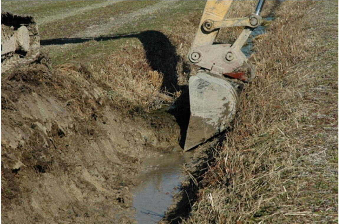
Illustration 3.3. Ditch dredging in Somerset County, Maryland. Spoil is typically spread near the ditch. (Courtesy Brian A. Needelman)
