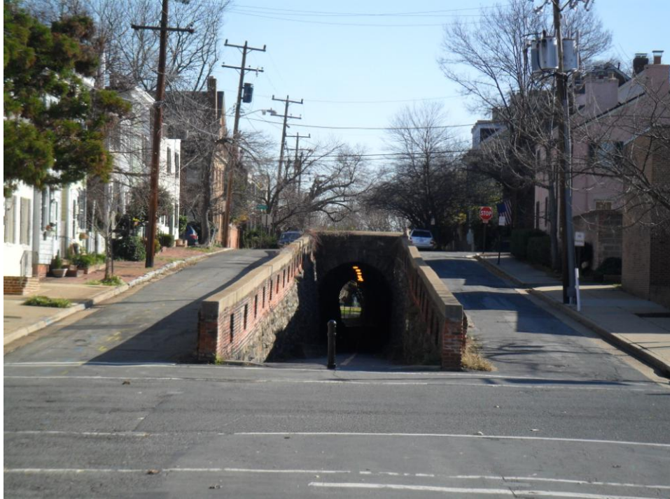
Figure 23: Wilkes Tunnel, site along the Hayti Trail, 2011
