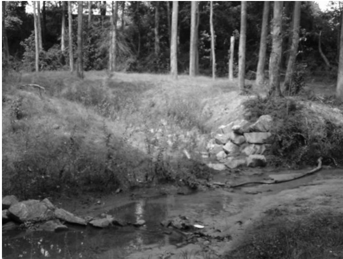
Figure 1.2. Photograph of a representative restored stream. Boulders have been placed on the channel banks to prevent bank erosion and have been placed in the channel to prevent channel incision.
