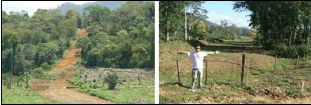
Figure 6. Early construction of the PETROBRAS natural gas pipeline slated to run through the range of the golden-headed lion tamarin in Bahia, Brazil. (photos taken by S. Zeigler, 2006)
