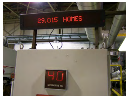
Fig. 23 Electrical control room .
