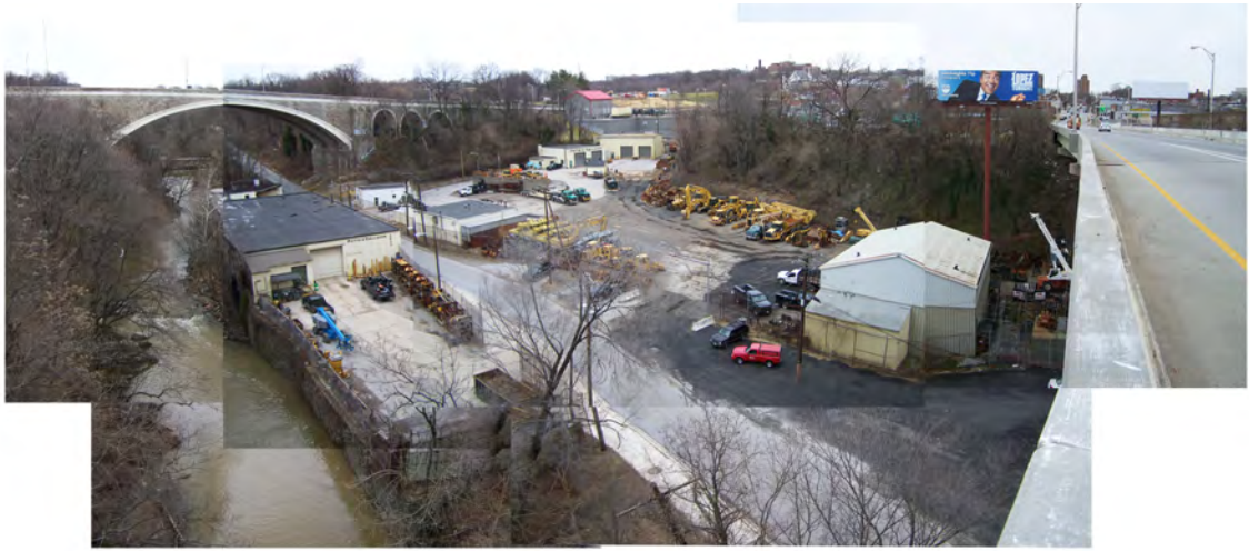
Fig. 5 Site Panorama from 28 th street Bridge.
