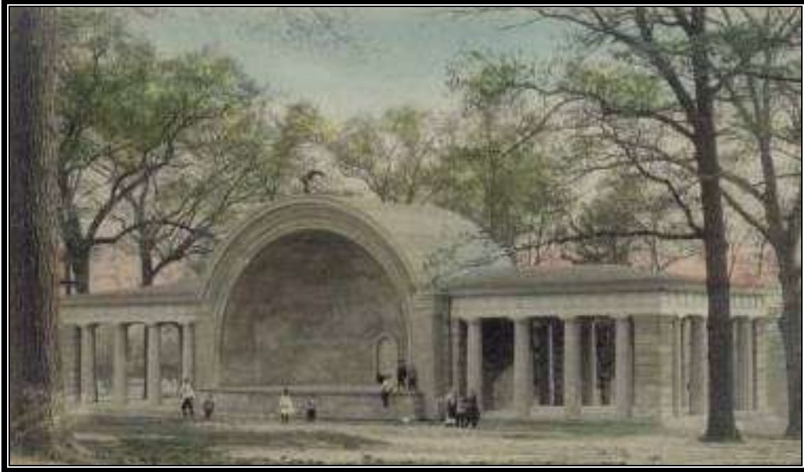
Figure 35: Bandstand at Clifton Park prior to 1947 fire. Courtesy of Thomas Paul.
