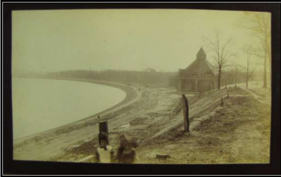
Figure 30: View of filtration plant and Clifton Reservoir with two children in foreground circa 1890. Courtesy of the Ferdinand Hamburger Archives, Sheridan Libraries, The Johns Hopkins University.
