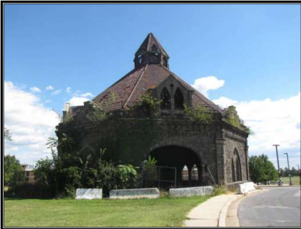
Figure 31: Valve House in September 2010. Facing southeast. Photo by author.
