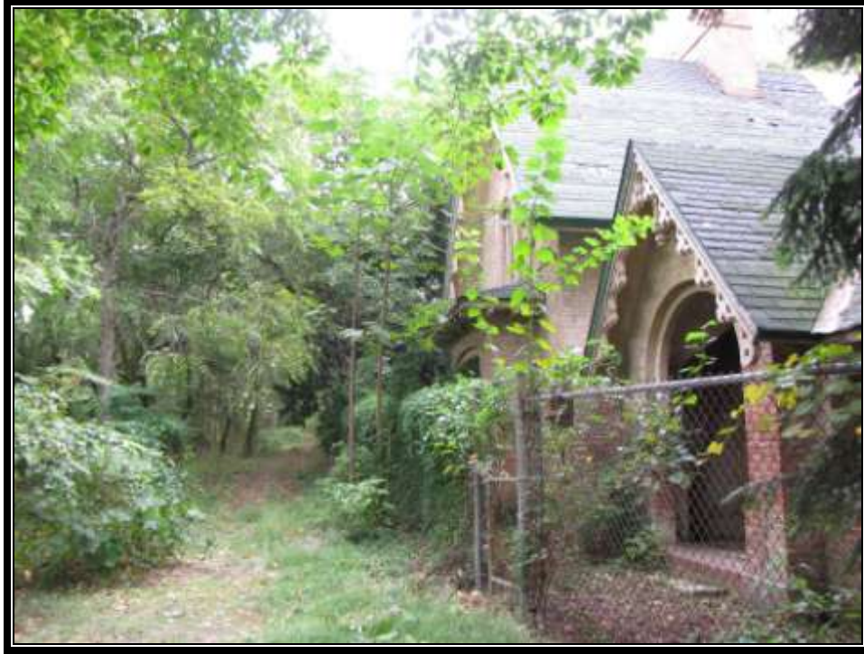
Figure 20: Gardener's Cottage September 2010. Photo by author.
