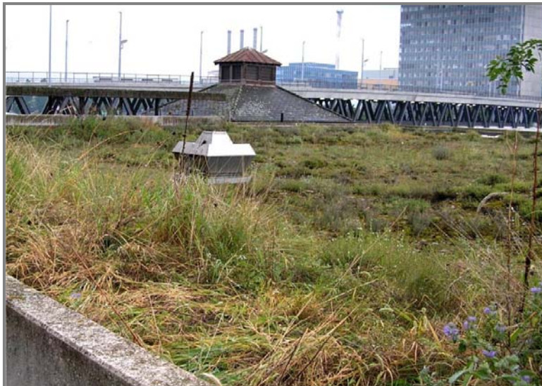
App. Fig. A2. After construction: green roof designed to attract ground-nesting and feeding birds. City of Basel, Switzerland. Source: Breinnsein, 2006.
