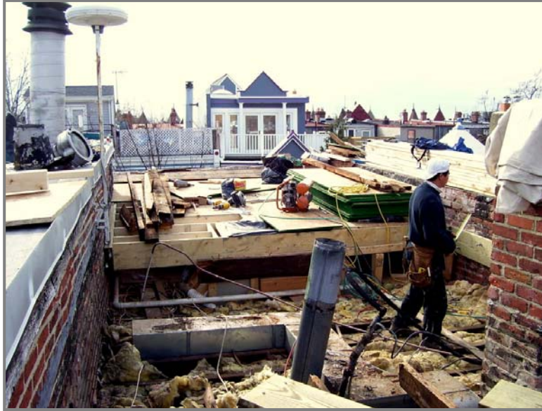
App. Fig. A3. Construction of a deck in the Flowers-Muller Residence. Project located in Adams Morgan, Washington, DC. Source: Capitol Greenroofs, 2010a.
