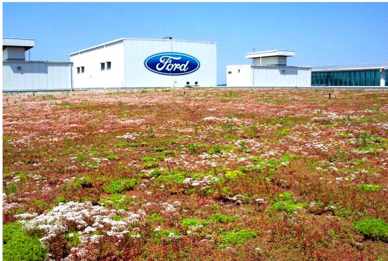
App. Fig. A10. Mature extensive green roof with Sedum species. Project located in Ford Motor Company's River Rouge Plant. Dearborn, MI. Source: greenroofs.com
