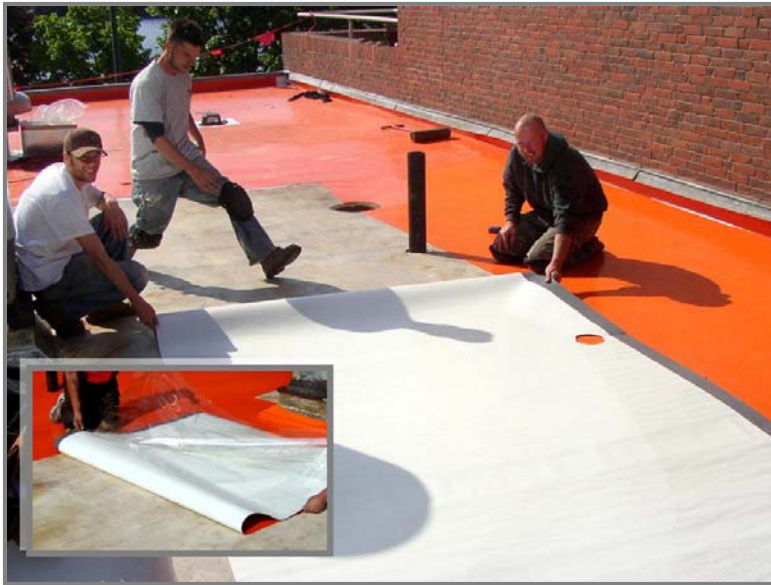
App. Fig. A4. Installation of a single-ply waterproofing membrane in Harvard University Institute. Project located in Cambridge, Massachusetts. Source: Capitol Greenroofs, 2010b.
