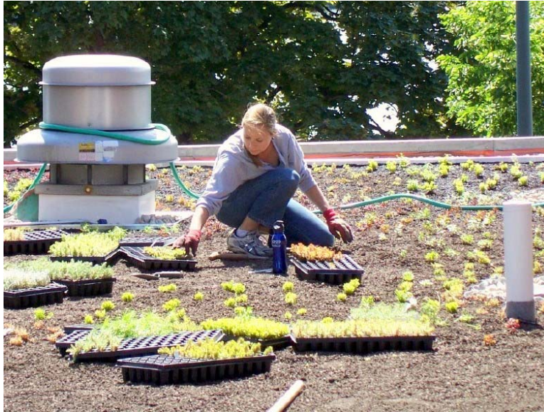
App. Fig. A9. Installation of Sedum species in Harvard University Institute. Project located in Cambridge, Massachusetts. Source: Capitol Greenroofs, 2010b.
