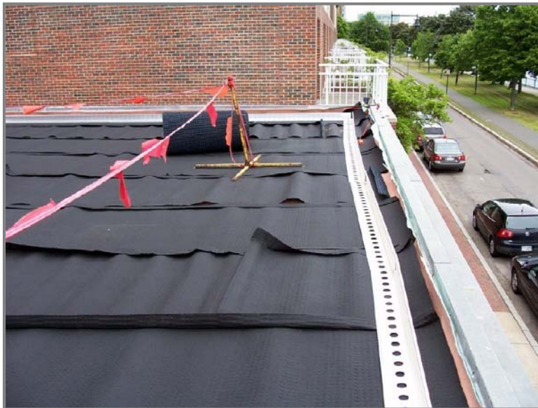
App. Fig. A8. Installation of a filter fabric in Harvard University Institute. Project located in Cambridge, Massachusetts. Source: Capitol Greenroofs, 2010b.
