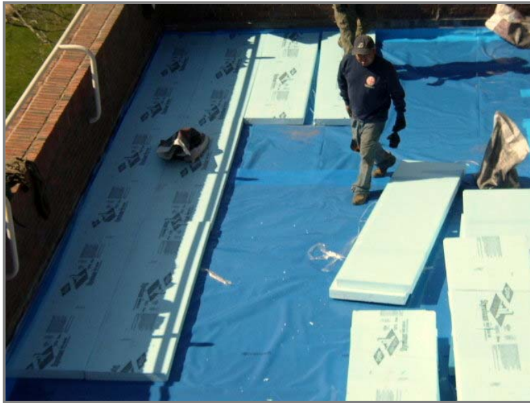
App. Fig. A5. Installation of insulating materials (Dow Styrofoam 40 lb density) in Harvard University Institute. Project located in Cambridge, Massachusetts. Source: Capitol Greenroofs, 2010b.
