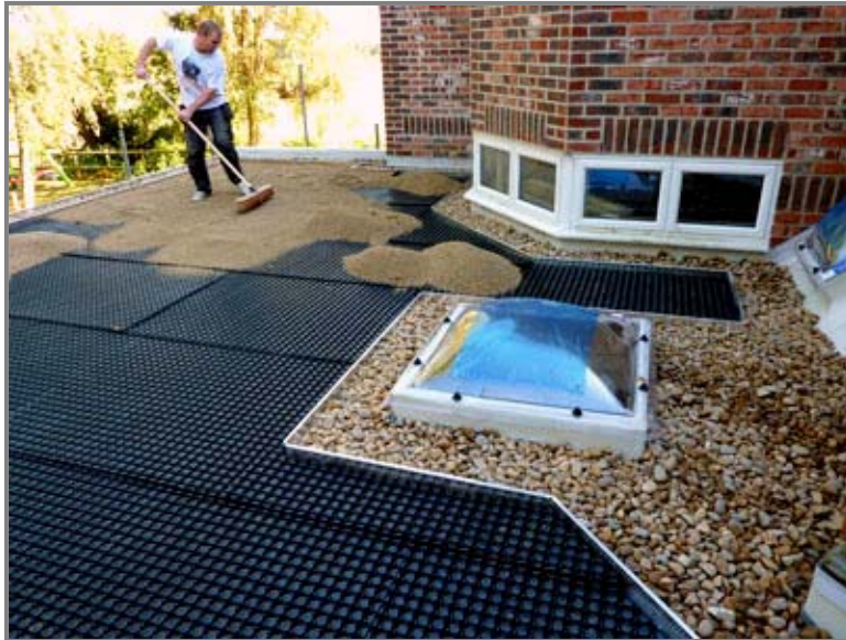
App. Fig. A7. Installation of a modular drainage layer. Source: Landmark Living Roofs Ltd, 2010.
