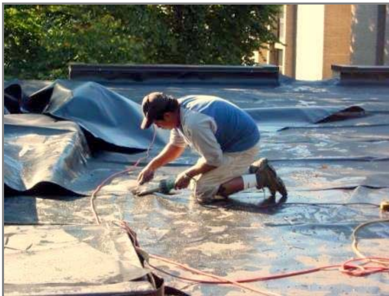
App. Fig. A6. Installation of a polyethylene root barrier in Harverford College, Pennsylvania. Source: Harverford College, 2010.
