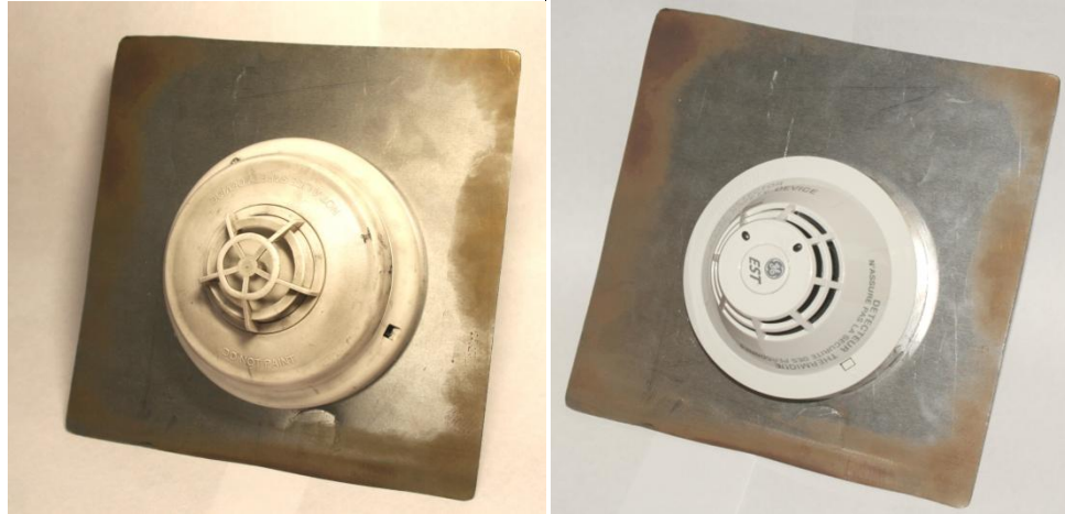
Figure 12 – Thermistor heat detectors mounted to their plunge plates. Detector B is shown on the left and detector D is shown on the right.
