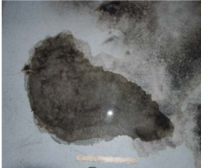
Figure 4-5 - Photo showing discoloration of the concrete pad from previous tests
