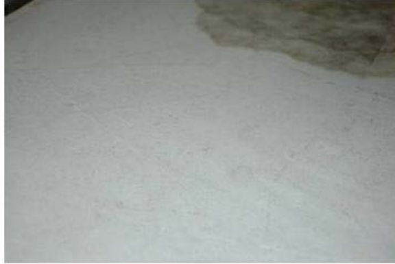
Figure 3-2 - Smooth texture of concrete pad used in testing
