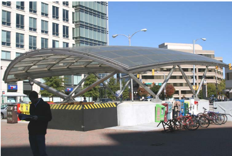
Figure: 2-1 – Washington D.C. Metro Entrance Canopy (Clarendon Station). Personal Photo 10.20.08.
