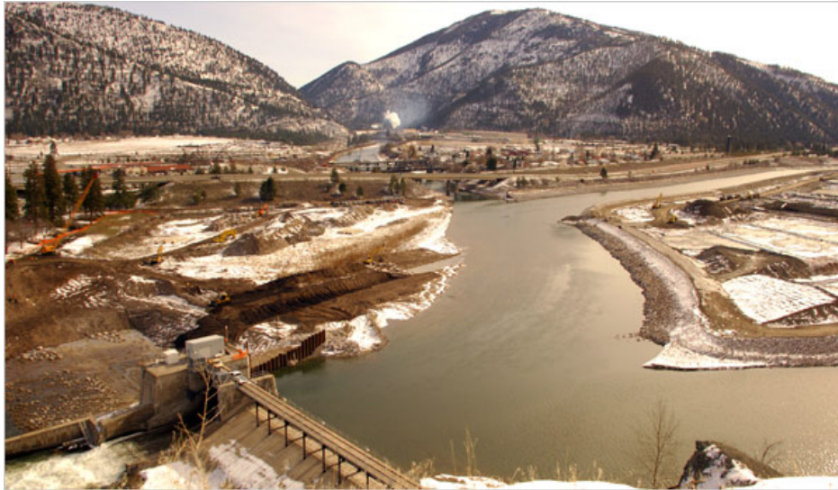
Figure 1. The 100-year-old dam is to be removed, and parts of the Clark Fork River will be re-joined.
