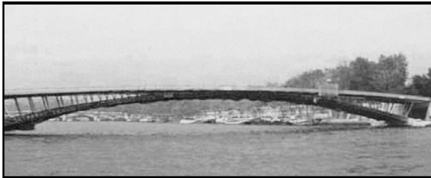
Figure 2.5: Pont du Solferino, Paris, France
