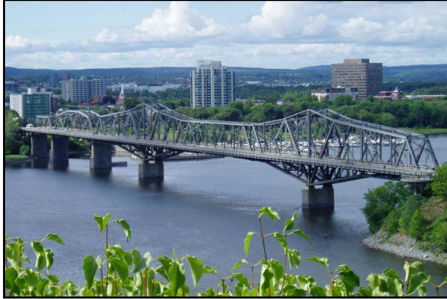
Figure 2.6: Alexandra Bridge, Ottawa, Canada
