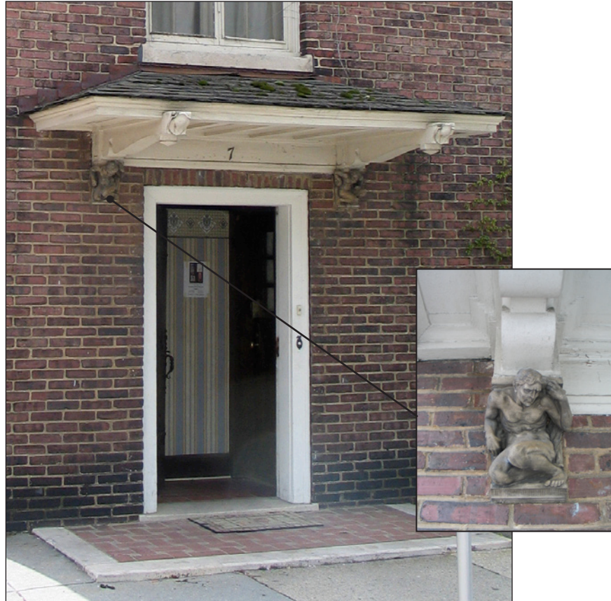
Figure 14. Sculptural cariatids by Schuler support the brackets of the hood over main entrance (Author)
