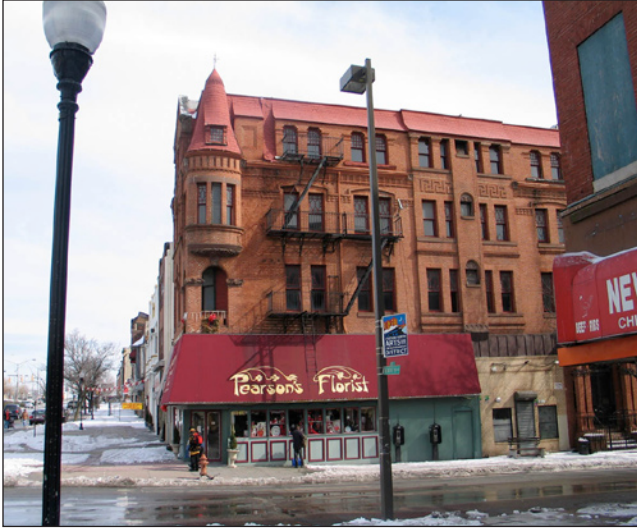
Figure 38. East corner of North Avenue and Charles Street showing the old Waldorf Hotel (Author)
