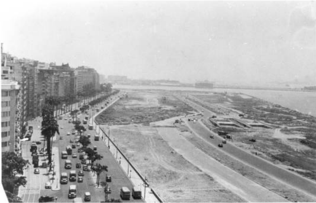
Figures 3.6 Aterro do Flamengo Construction in the Early 1960s
