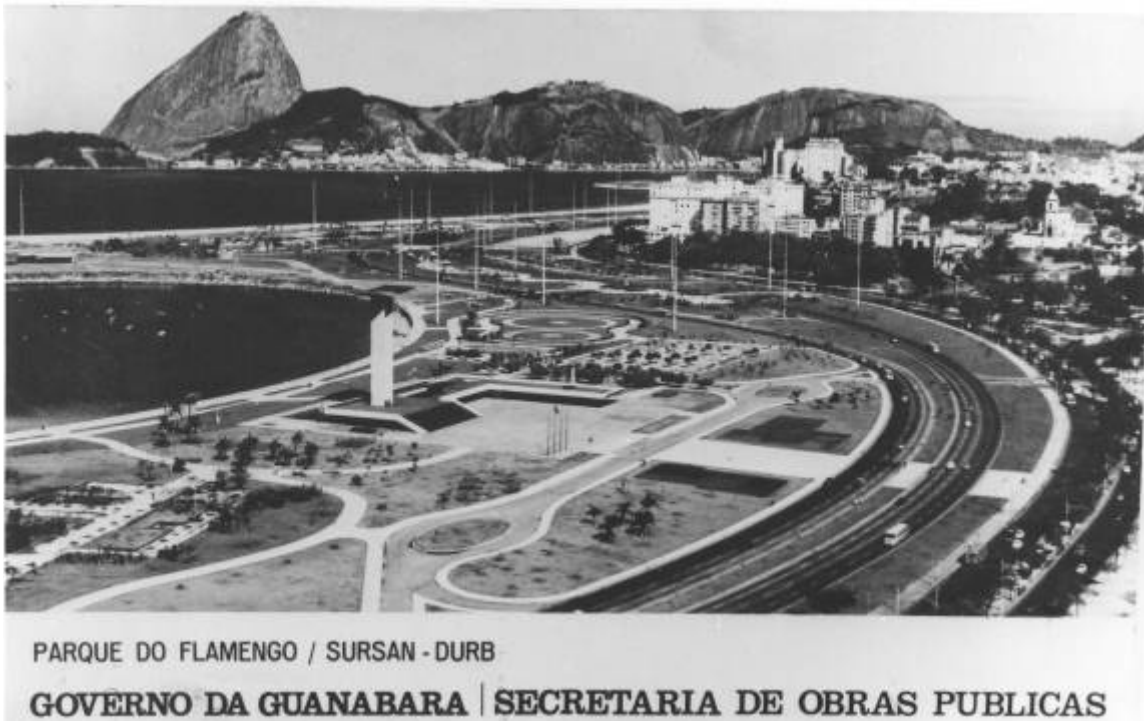
Figure 3.9 Completed Aterro and Parque do Flamengo – Mid 1960s
