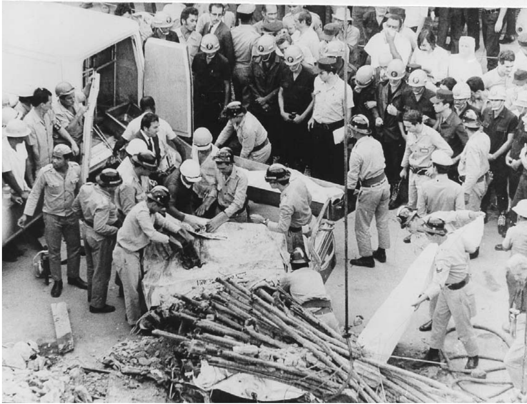
Figure 7.6 Injured and Killed Victims from the Collapse
