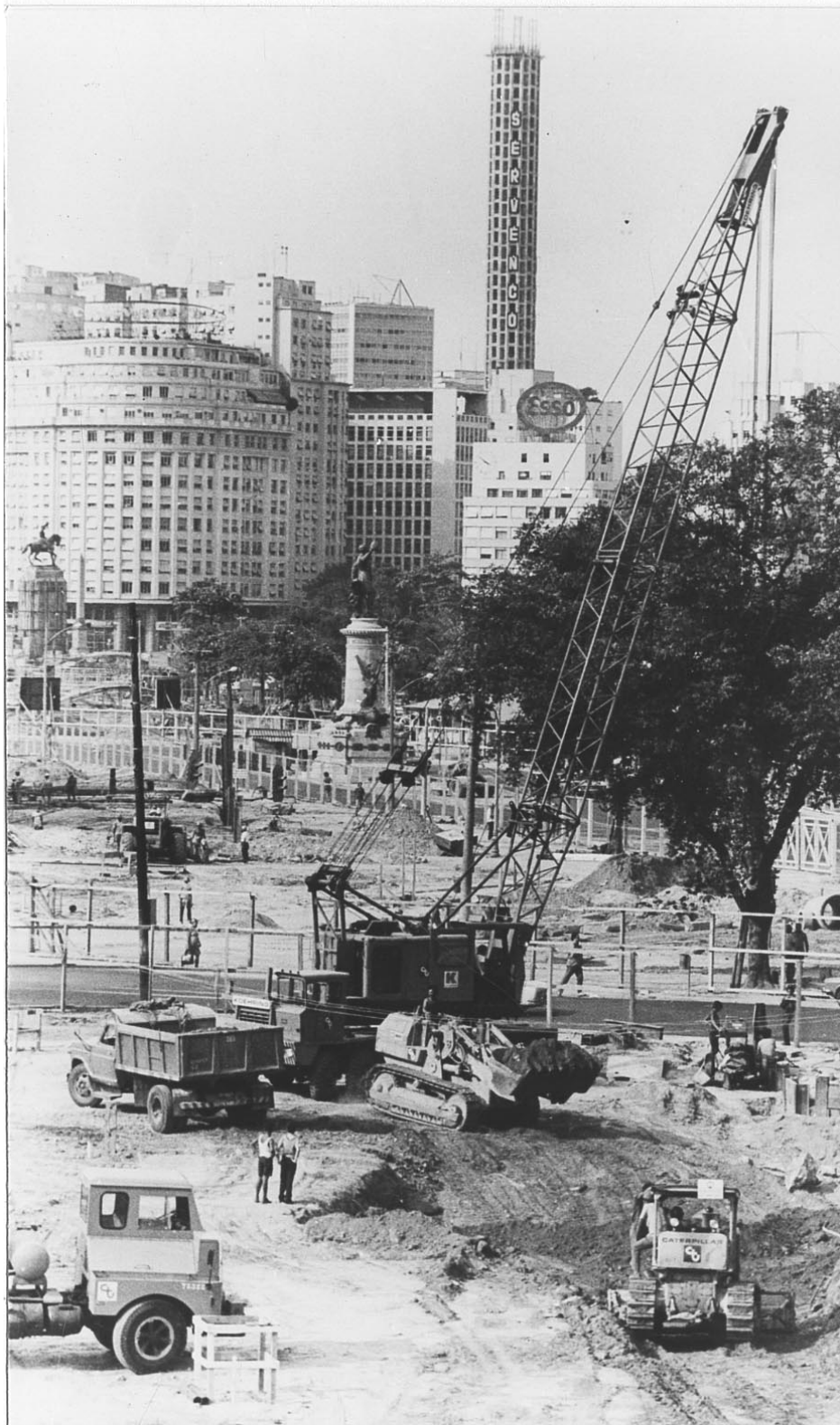
Figure 7.7 Construction of the Metrô in the Early 1970s in Downtown Rio
