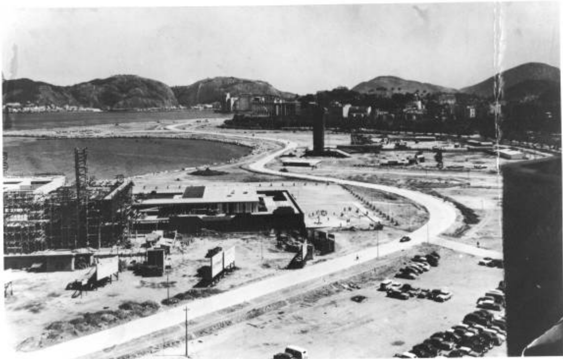
Figure 3.7 – Construction of the Aterro do Flamengo and Museu da Arte Moderna
