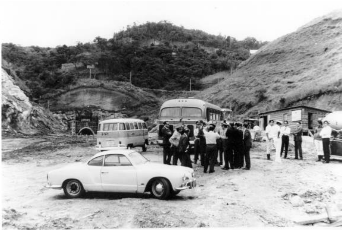
Figure 5.2 Construction Beginning on the Túnel Joá
