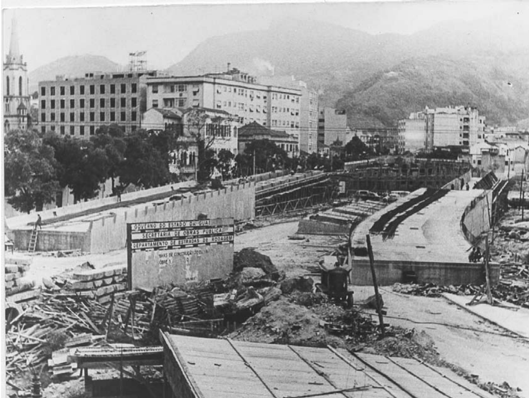
Figure 7.1 Construction of the Elevado Paulo de Frontin
