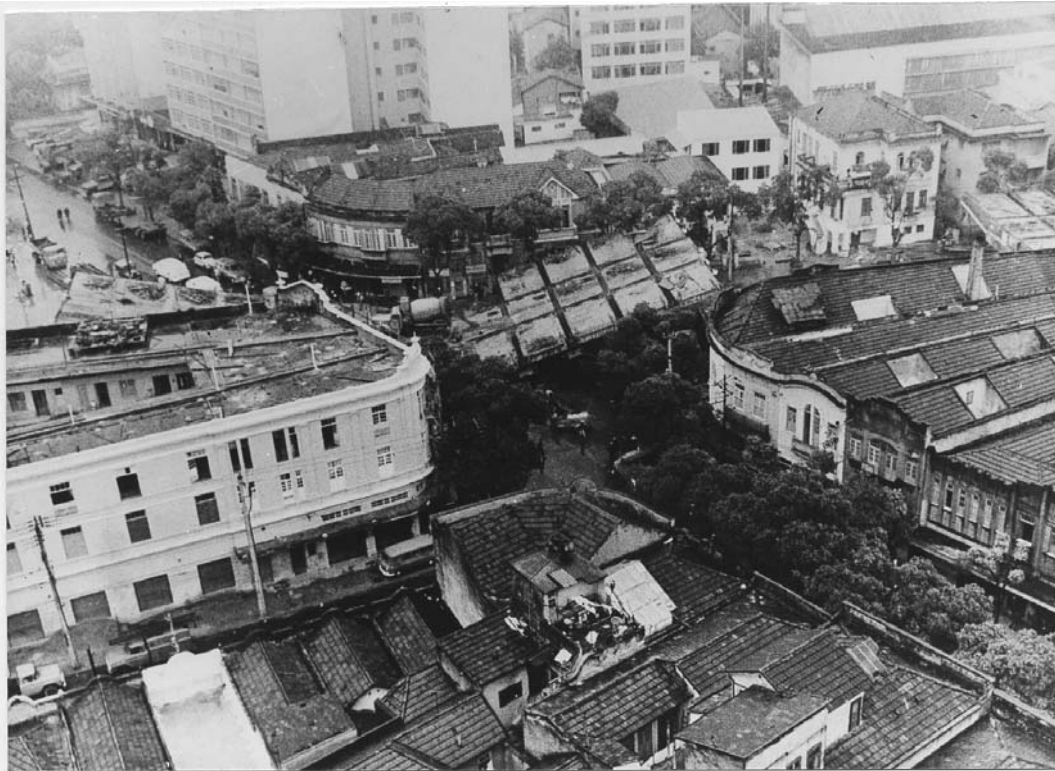
Figure 7.3 Collapse of the Elevado
