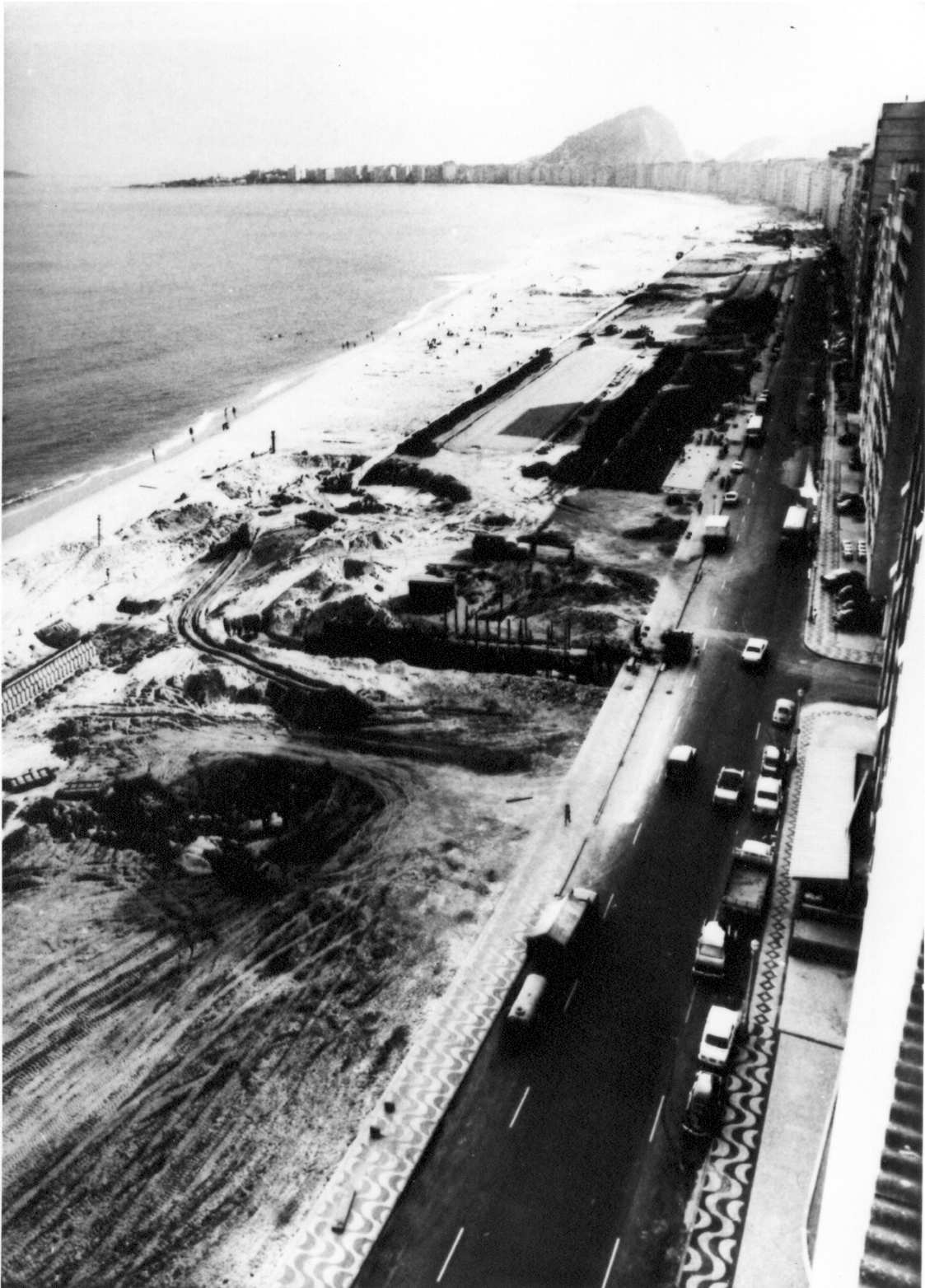
Figure 5.9 The Building of an Additional Lane along the Avenida Atlântica
