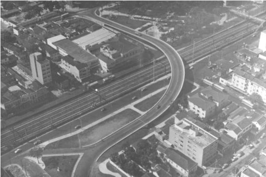
Figures 5.1 – The Viaduto do Méier Facilitating Connections for Cars
