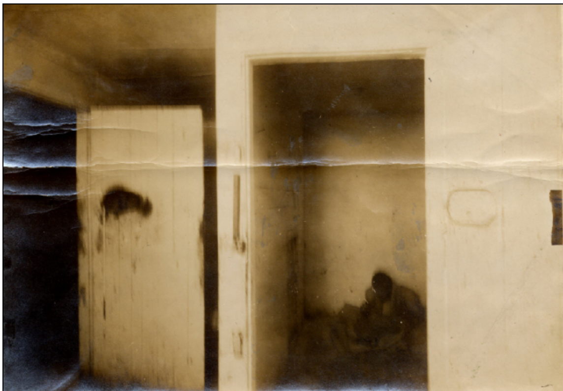
Figure 9. Basement cell, Kent County Almshouse, African American building, 1908 (Maryland State Archives).
