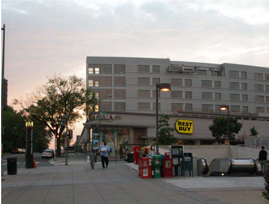
Figure 35: Tenleytown Metro Stop East Side view looking West—the entrance is evident by the cluster of newsstands and the uncovered escalators.
