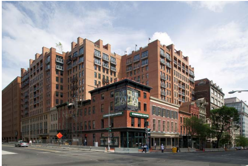
Figure 68: The Jefferson at Penn Quarter —displaying one of the densest housing structures in downtown Washington (616,000sf composed of 35,000sf of retail and about 428 apartments). Although it comprises this density, its massing doesn't overwhelm the street. On the contrary, the housing has been skillfully set back from the three and four story buildings, not only to allow the historic buildings to be read in their full form, but to create a more human scale and to allow more sunlight to reach the street.
