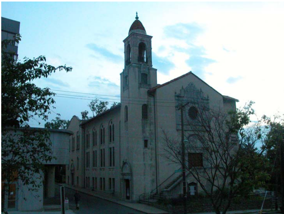
Figure 29: Eldbrooke Methodist Church —on River Road behind the 'Cityline' Condominiums
