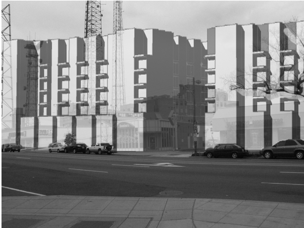
Figure 101: Wisconsin Avenue Montage
