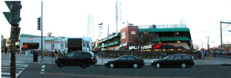
Figure 13: South Elevation of site (Albemarle Street) —showing the one and two story buildings on the West, and the three story parking garage and grocery store divided by an alley. The Metro station entrance is almost invisible, marked only by a kiosk and a large number of newsstands. The radio towers on the Northern horizon contribute to visual clutter, and the low hedges and solitary tree don't do much to relieve the disorder. A taller building would mostly conceal the towers from this angle.
