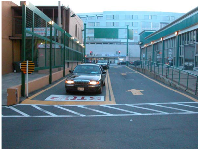
Figure 19: View of internal alley looking towards Wisconsin Avenue —the alley is intended as a thruway to the grocery store's parking garage. Note the safety features for pedestrians, such as the painted crosswalk and STOP sign, as well as the railing placed on the sidewalk edge, due to the somewhat dangerous configuration of the alley.
