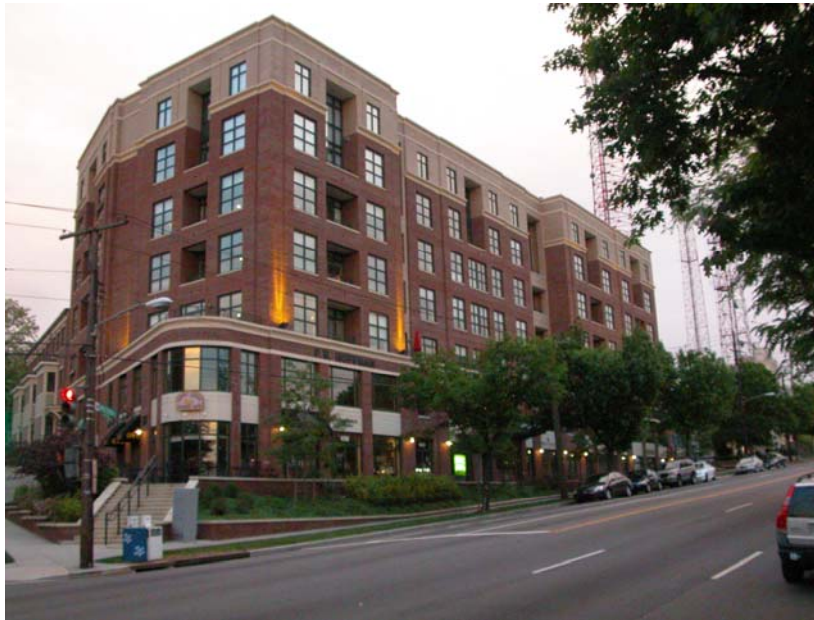
Figure 17: “Tenley Hill” Housing and Retail —located on the East side of Wisconsin Avenue, two blocks north of the Site, and completed in 2000. The expensive and quickly occupied structure negotiates the steep grade with a two-story retail and office base.
