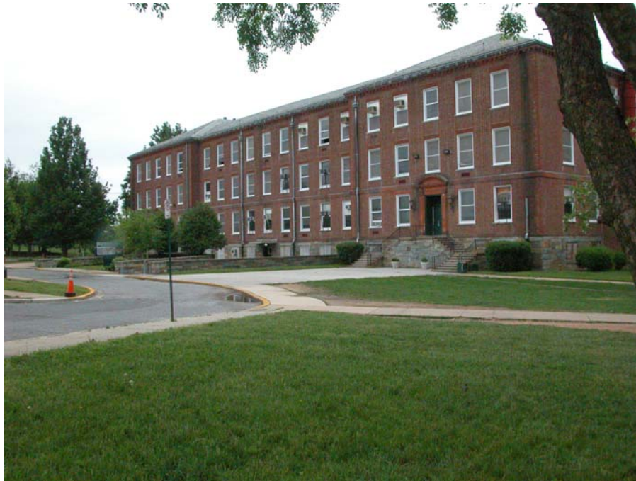
Figure 27: Woodrow Wilson Senior Public High School —located across the street and East from the site block.
