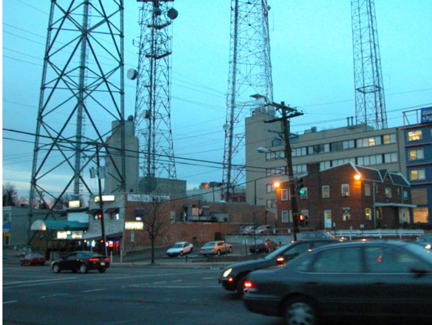
Figure 30: Radio Towers —Street level view from Wisconsin Avenue and Brandywine Street. The towers are placed unusually close to the sidewalk. The closest in View, was intended for HDTV broadcasting, but, unfortunately was not completed due to pending litigation. The concrete cylindrical structure is known as Tenley Tower built in 1947 by the Western Union Telegraph Company. During the Cold War, it was a relay point for national security networks. 22
