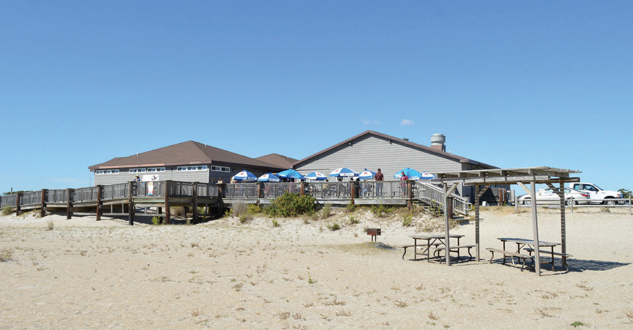
EXISTING DAY USE BUILDING BUILT IN 1990
