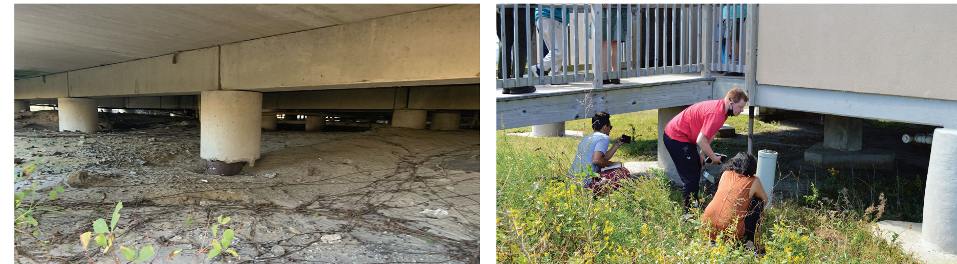
STUDENTS DOCUMENT EXISTING FOUNDATION DURING SITE VISIT
