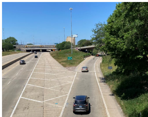
Figure 44: View from Wentworth overpass toward the embankment. Stored rail cars are visible but other views are obstructed.
