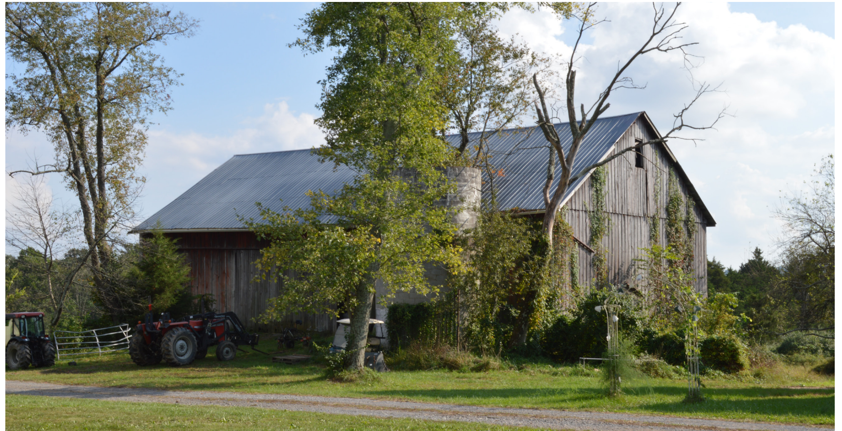
Existing bank barn (Evan Lipka)
