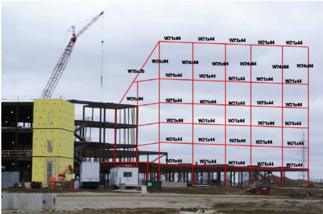
Figure A.86: The process for the engineers with augmented reality [73] to design a building with data visualization
