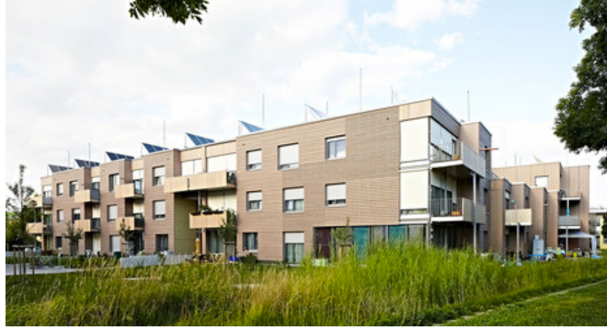
Figure 0.1 Hollerstauden residential building, view from southwest
