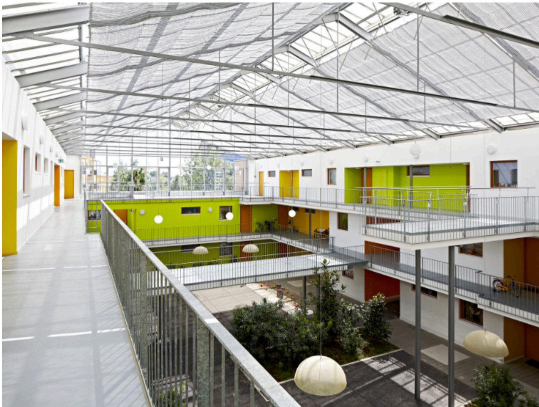
Figure 0.3: Exterior and interior views, showing the atrium.
