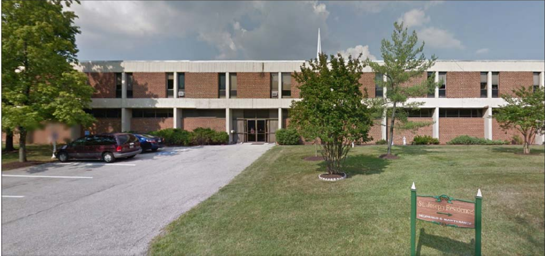
Figure 26: Front Façade Photo by Good Shepard Services
