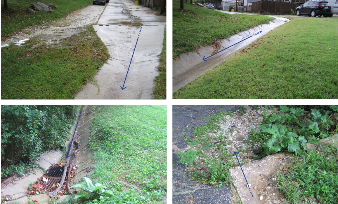
Figure 20. Existing conditions—concrete drainage channel
