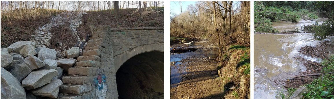
Figure 22. Existing conditions—Remington Avenue bridge and Stoney Run stream
