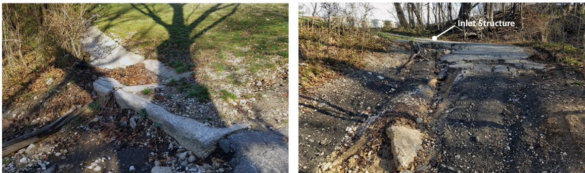
Figure 21. Existing conditions—storm sewer inlet structure and asphalt road
