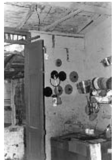
Figure 32. Kitchen. These tiny spaces are shared by several families [atelier d' architecture de Medellin]
