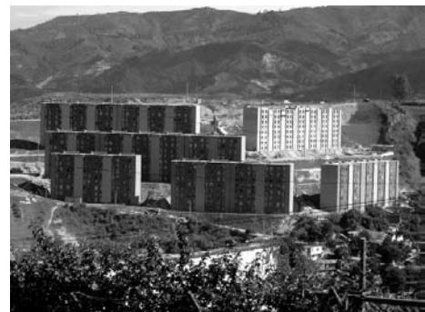
Figure 2. Low-income project in San Cristobal , Medellin. Repetitive high rise pattern houses do not represent variety of life-styles [author]
