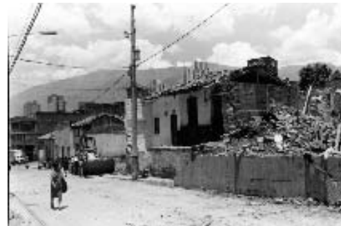
Figure 24. Physical deterioration. Demolished shacks and empty lots are another pathology found in Niquitao. [atelier d' architecture de Medellin]
