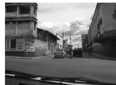
Figure 20. Carrera 44 "Niquitao". N-S Most deteriorated road. [author]
