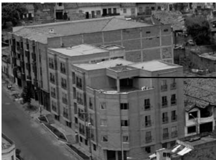
Figure 28. Corvide housing projects. These projects are the latest generation of housing projects in Niquitao. Notice treatment of sidewalks [author]
