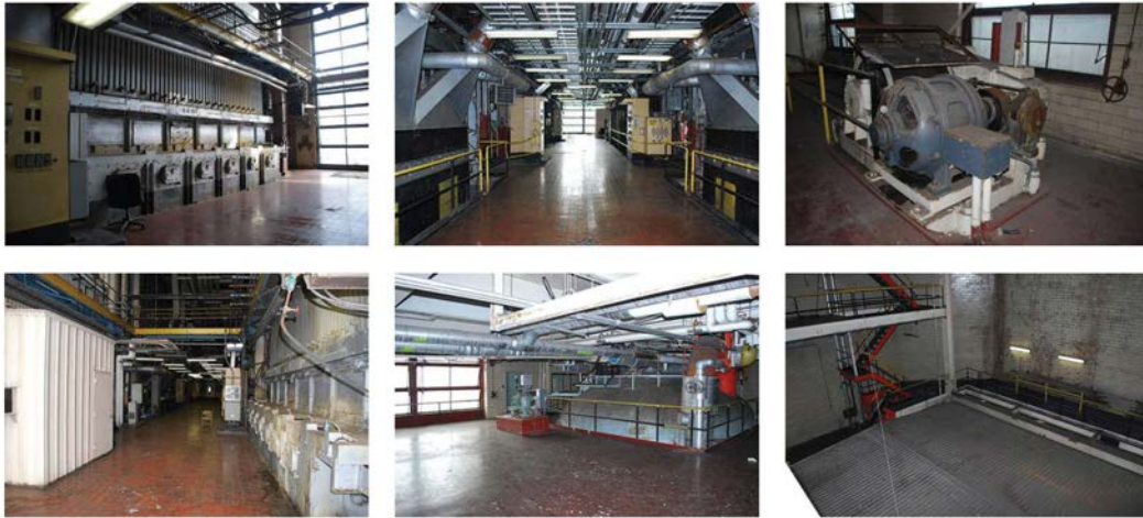
Figure 15 – Interior views in current condition
