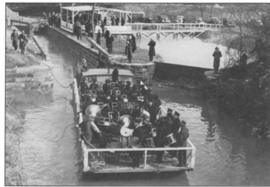
Figure 5 – 1939 photo of the dry dock, filled with water [Mackintosh, 34].
