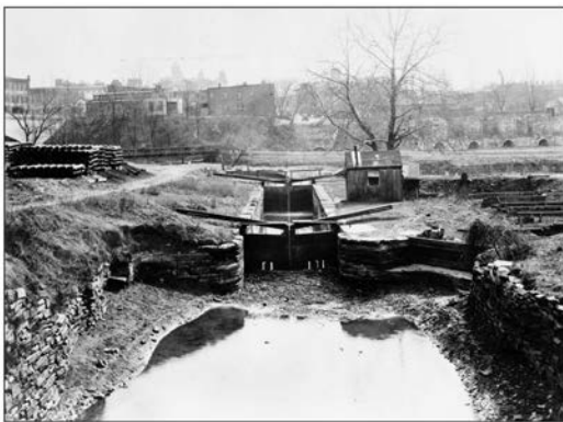
Figure 4 – 1910 photo of the dry dock with boat supports visible [LeeDecker and Kuhn, 44].
