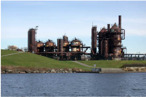
Figure 35 – Seattle's Gasworks Park [http://www.seattle.gov/tour/union.htm]
