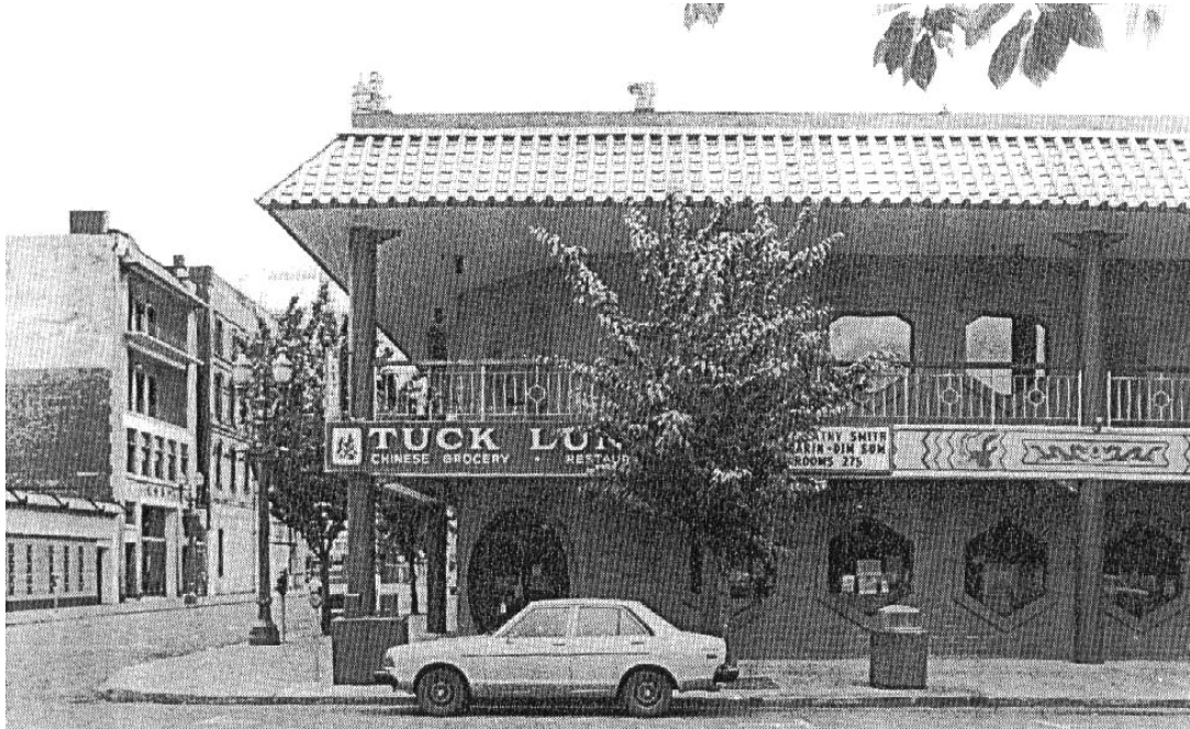
Figure 51. Tuck Lung Grocery and Restaurant (1977) in Portland's Chinatown attempts to portray 'authenticity' of Chinese culture through elevation. Its disneyesque appearance only reflects the true use of the building-a tourist attraction. (Chinatown Historic District)
