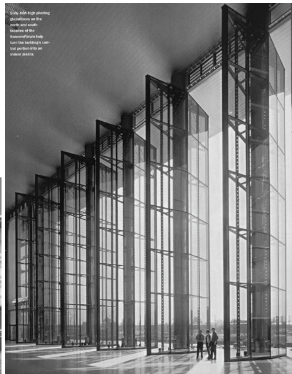
Figure 89 Autostadt façade opens great piazza (Weber-Hof)
