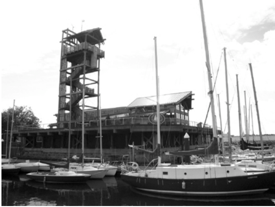
Figure 20 Existing Living Classrooms center on north edge of site
