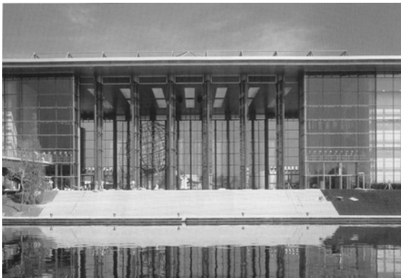
Figure 88 Autostadt glass façade and grand stair (Weber-Hof)
