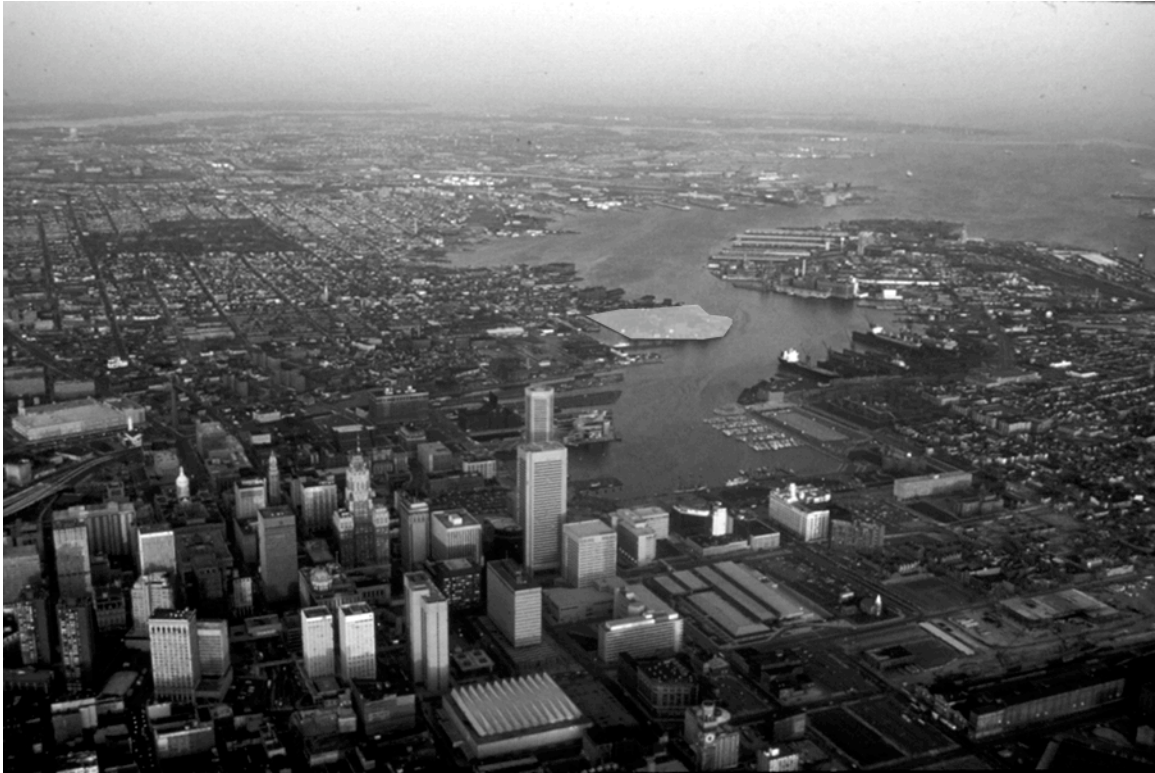
Figure 48 1980's Aerial: prominence of site on waterfront (Landslides)
