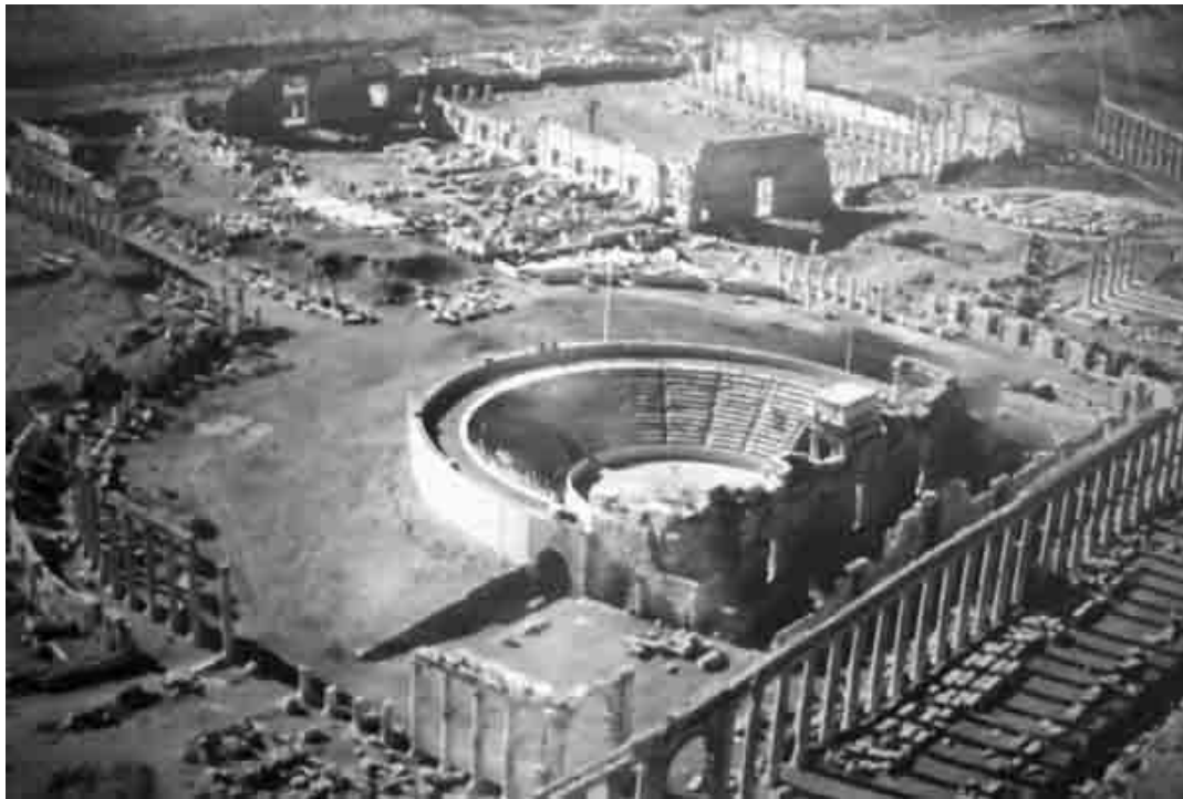
Figure 11: Aerial view of the restored theater and of the agora looking west (photograph by Waleed al-As'ad)
