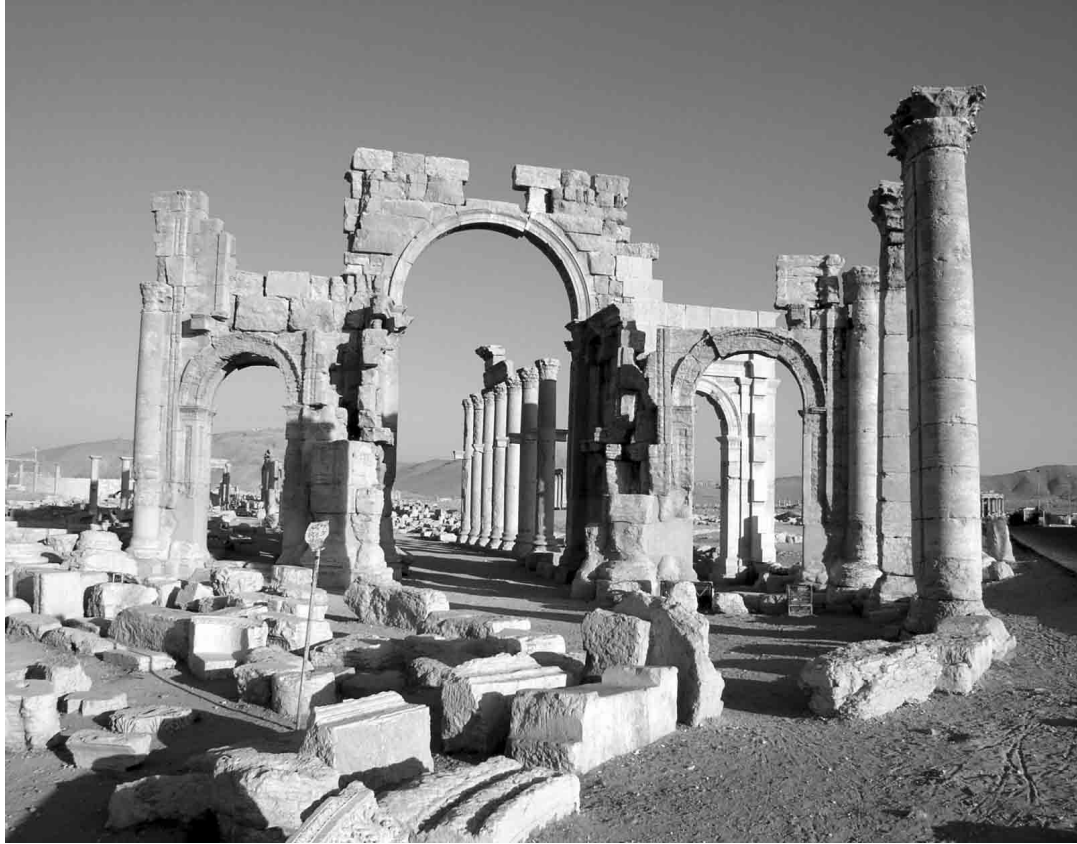
Figure 13: Monumental Arch looking northwest. The arch masks a sharp bend in the colonnade.
