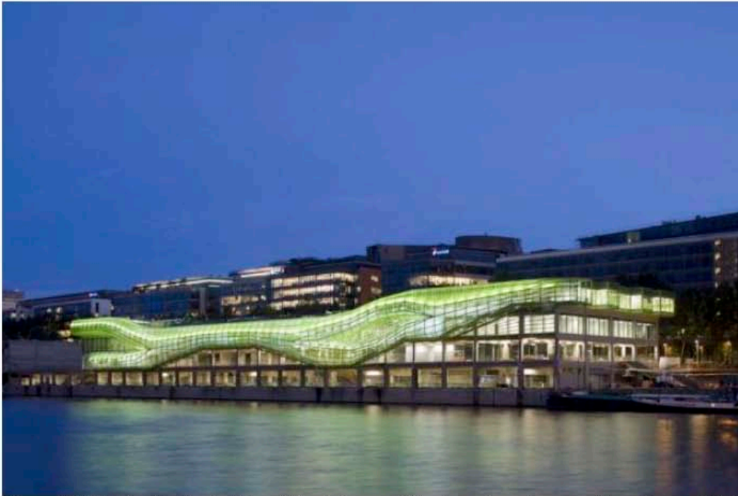
Figure 20 Docks De Paris City of Fashion and Design showing new façade overlaid over existing concrete building [ www.contemporarist.com ]
