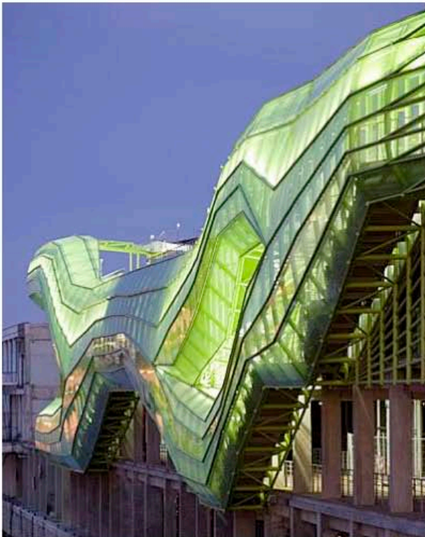
Figure 21 Showing thickened façade [ www.contemporarist.com ]
