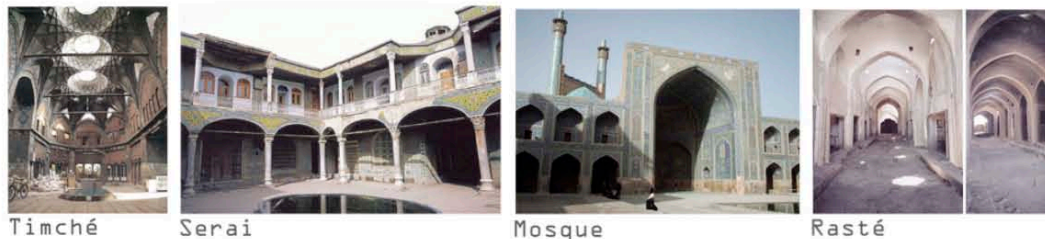
Figure 54 The four main spatial elements of the bazaar: The Timché, The Serai, The Mosque and the Rasté. [image provided by author]
