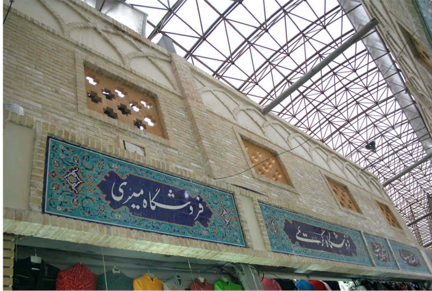
Figure 48 Tajrish Bazaar: Restorations have included adding skylights and trusses, replacing the old brick facades, and the addition of the newer signs with Persian motifs
