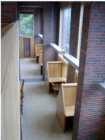
Figure 19 A good example of an inhabitable skin where the reading carrels are embedded within the load –bearing façade to make use of the light as well as the view [www.designlaboratory.com]
