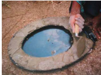
Figure 5-8: Plastic toilet seat filled with strong concrete
