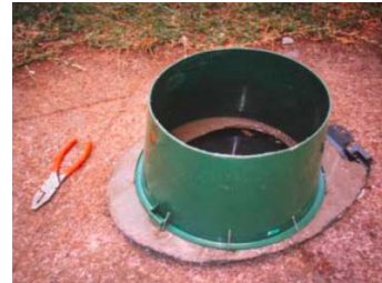
Figure 5-9: Plastic bucket placed over toilet seat
