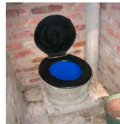
Figure 5-12: Completed low cost pedestal with plastic seat
