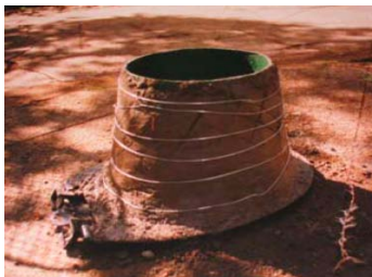
Figure 5-10: Concrete reinforcement added around first layer of concrete
