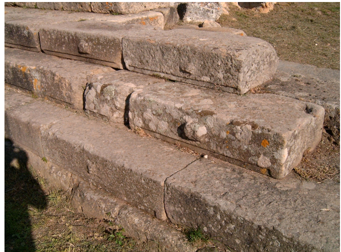
The stylobate of the Hellenistic temple, showing the tenons still on the stones. (Author's photo)
