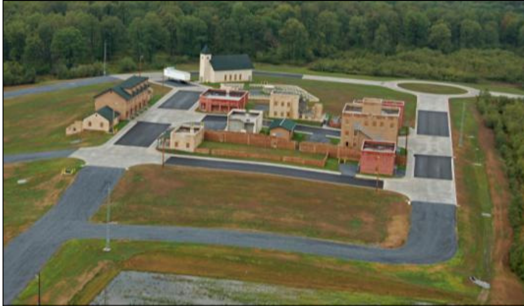
Figure 4.19: Aerial photograph of Fort Indiantown Gap site provided by the Army Research Lab.
