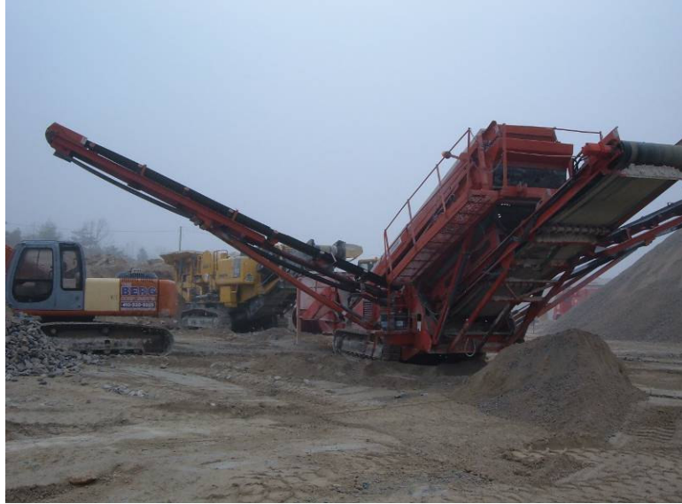
Figure 3.1 Crusher Used to Produce CCA at the Concrete Plant
