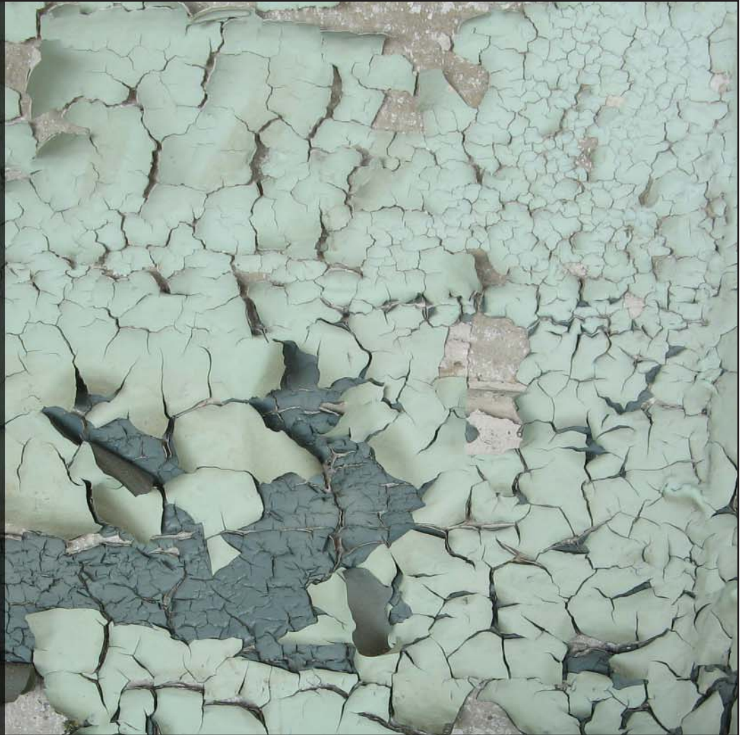
Figure 43: Peeling Lead Paint on a Column. Lead paint is everywhere in these old buildings, and the crunch of paint flakes underfoot is incapable. Paint clean up may pose a greater challenge than the asbestos simply because it is everywhere. [Photograph by author.]
