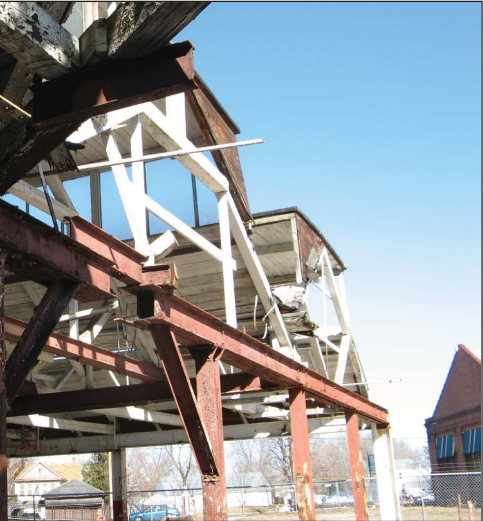
Figure 36: Building 7 Damage. This photograph shows the building with one of the most severe levels of damage including collapsed building sections; most of the wooden clerestory windows in this building are also glassless and rotting away. [Photograph by author.]
