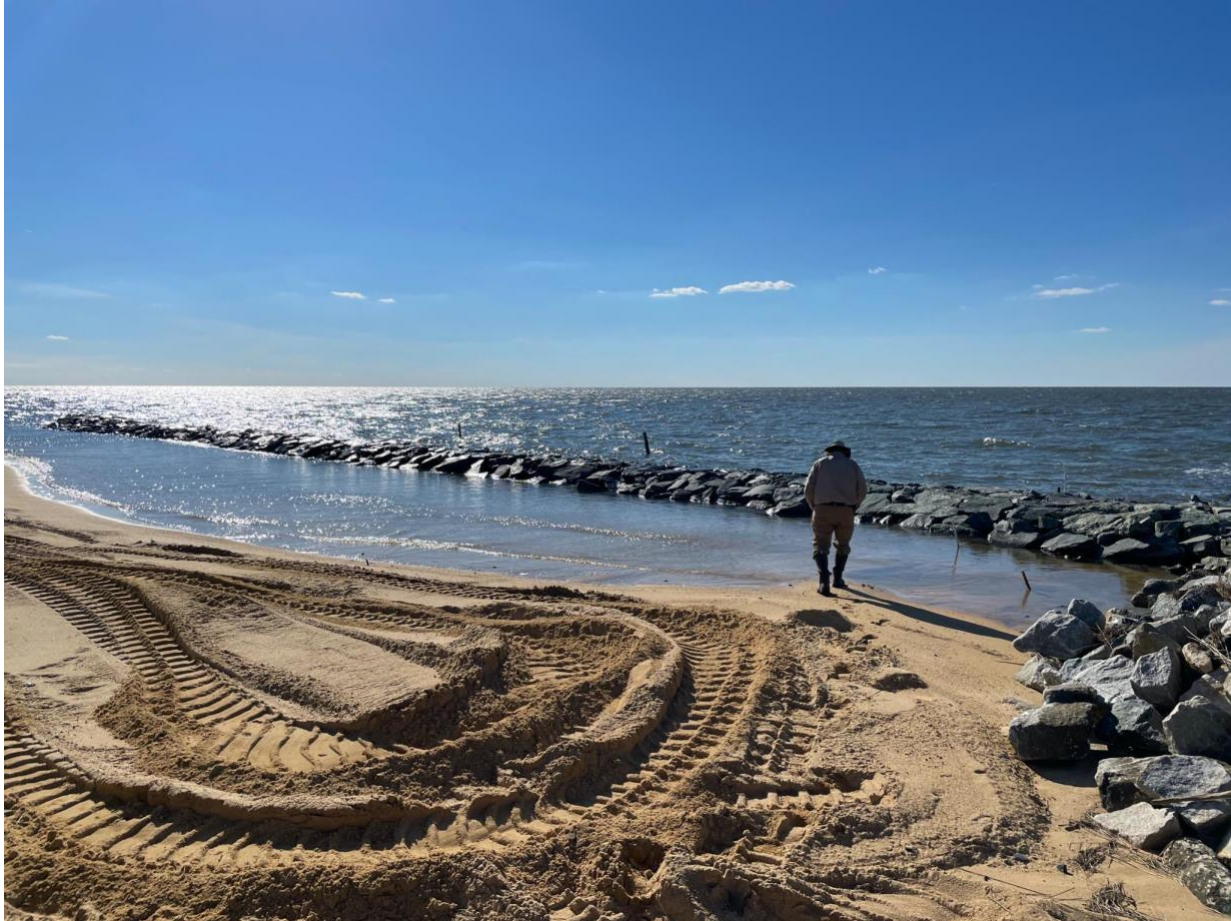
Rip-rap on the breakwater to protect the Deal Island Peninsula from more flooding. The project brought the news media to the island, but they didn't focus on Dames Quarter. Photo: Rona Kobell
