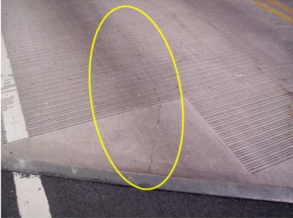
Figure 3-3: Longitudinal Crack on the Top Surface of the Knoxville Bridge.
