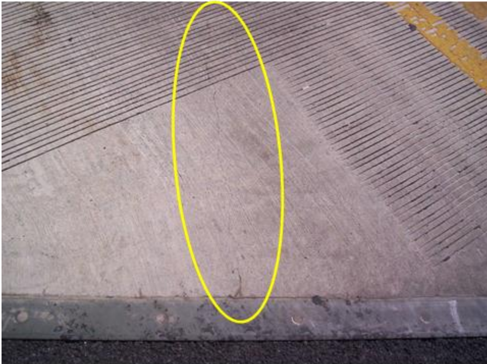
Figure 3-2: Longitudinal Crack on the Top Surface of the Knoxville Bridge.
