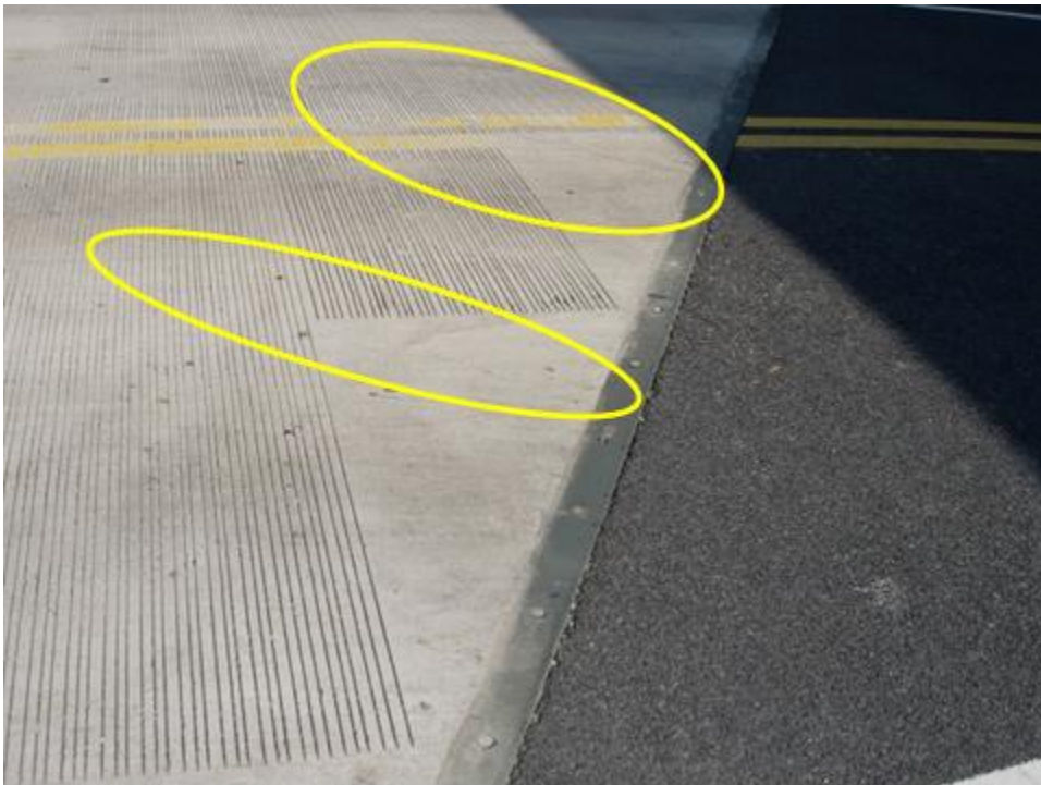
Figure 3-4: Longitudinal Cracks on the Top Surface of the Knoxville Bridge.
