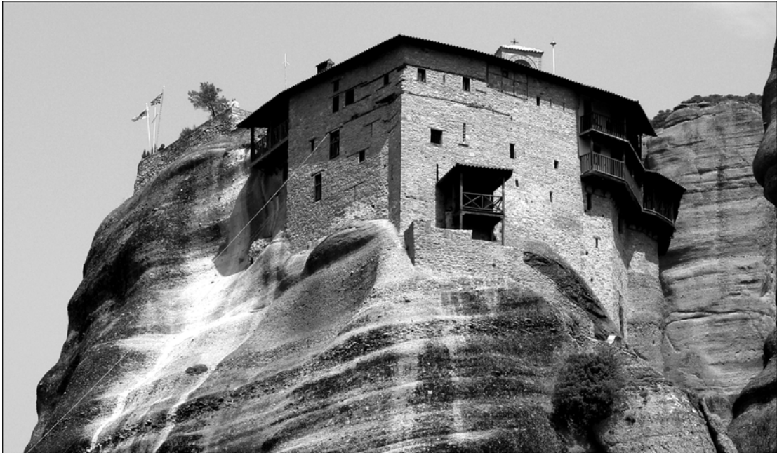
The Monastery of Agios Nicolaos Anapausas (#24) is the purest example of a ledge construction in Meteora, in that it is not situated at the summit of the rock but on the side.
