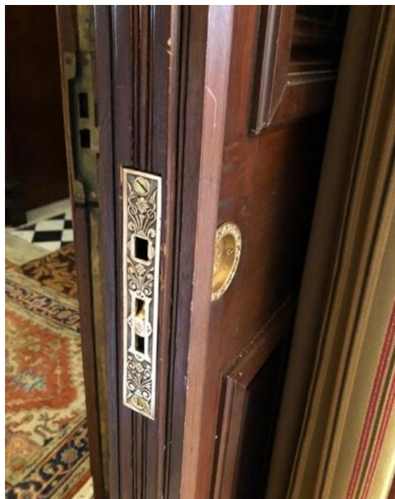
Figure 12. Old Korean Legation Building. Door hardware. 1500 13 th ST NW, Washington D.C.
