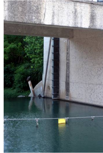
Figure 71: View of steel doors that shut during flood stage to protect the Paseo del Rio from flood damage.
