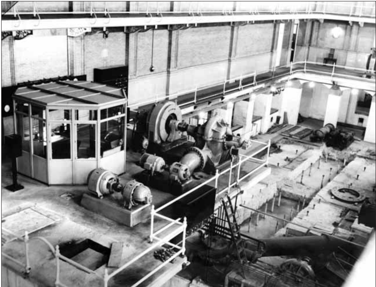
Figure 13: Main pump room, circa 1950
