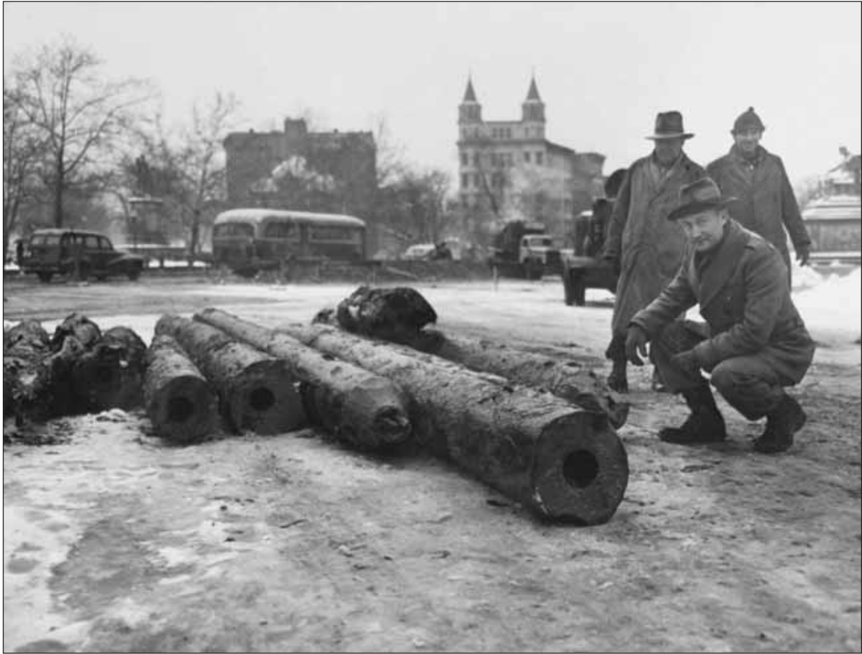
Figure 4: An early water pipe made from bored logs Staff Photographer, Washington Star , Untitled (Log Pipes, February 5, 1948) . © Washington Post , used with permission
