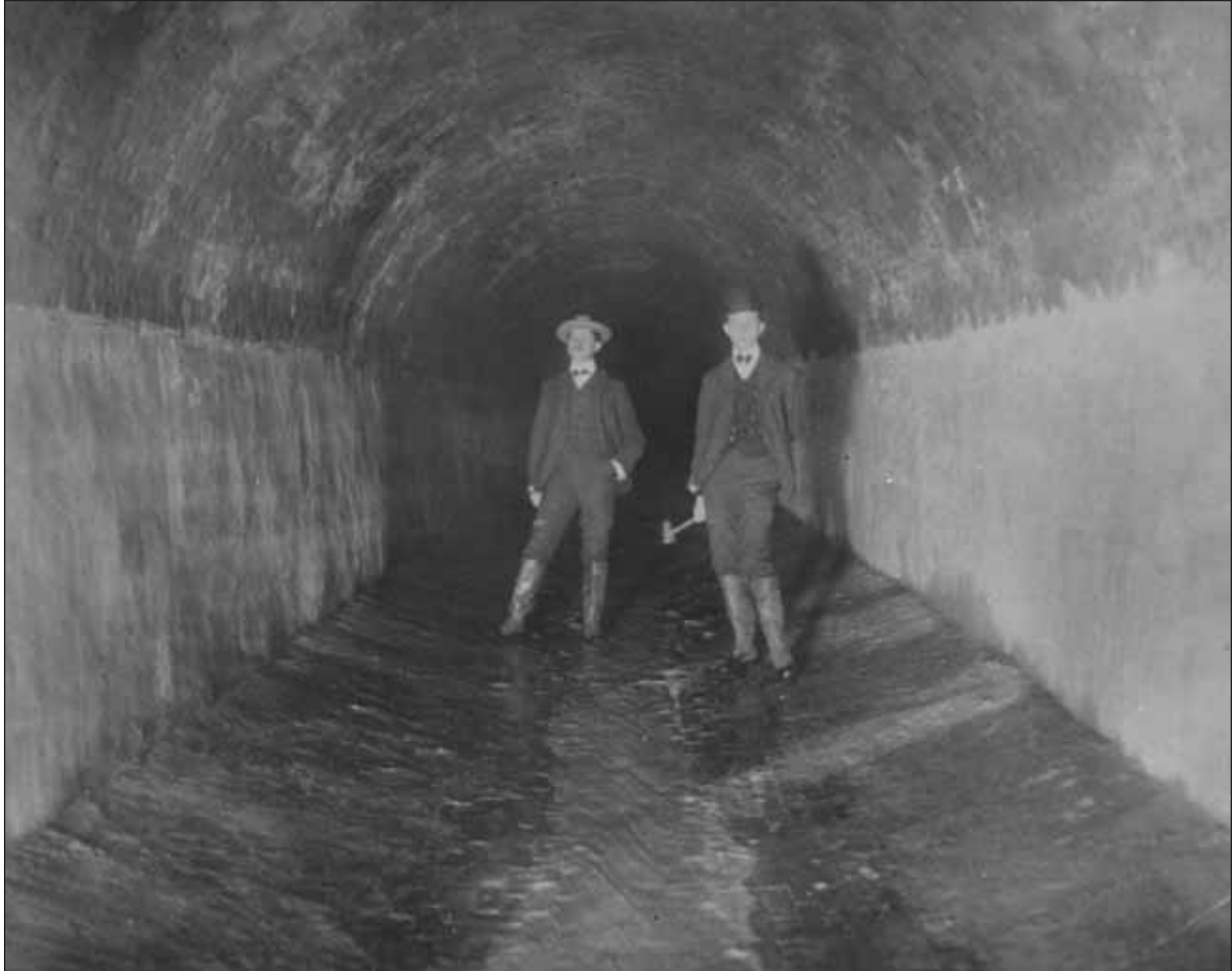
Figure 7: Workers in the Lydecker Tunnel, circa 1900 Staff Photographer, Washington Star , Lydecker Tunnel . Original Caption: "Tunnel lining showing plastered stone sidewalls" © Washington Post , used with permission
