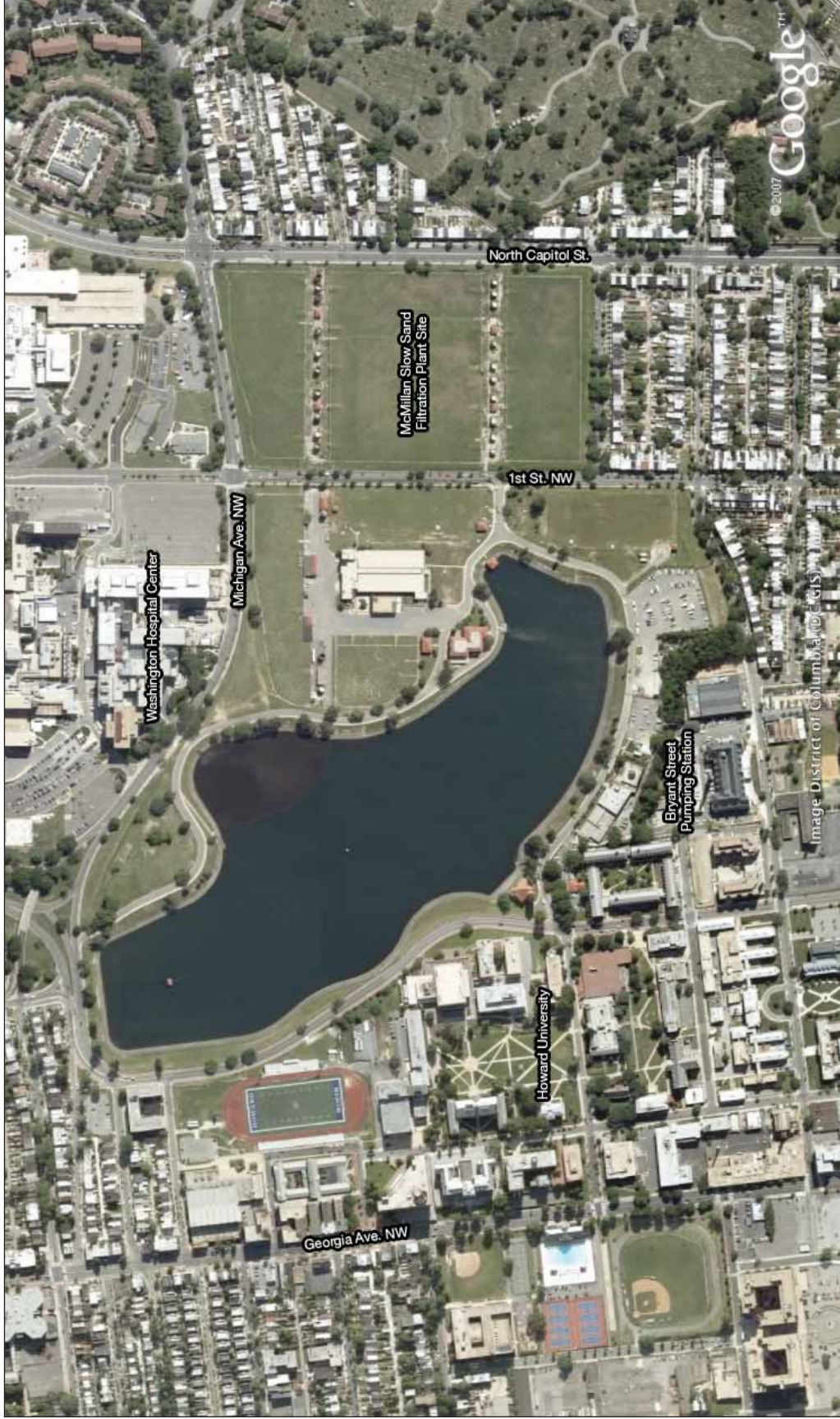
Figure 2: Aerial photograph of the Bryant Street Pumping Station and surroundings Google Earth, 301 Bryant Street NW, Washington, D.C.
