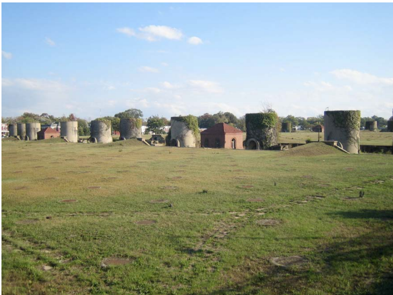
Figure 68 McMillan Sand Filtration Plant visible from North Capitol Street. http://upload.wikimedia.org/wikipedia/commons/e/e9/McMillan_Sand_Filtration.JPG
