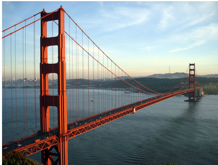
Figure 2 – Golden Gate Bridge completed in 1937 7
