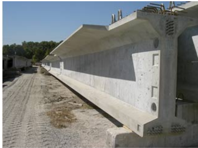
Vapor cured bulb-T-members await transport and final installation on Atlanta Hartsfield's fifth runway project
