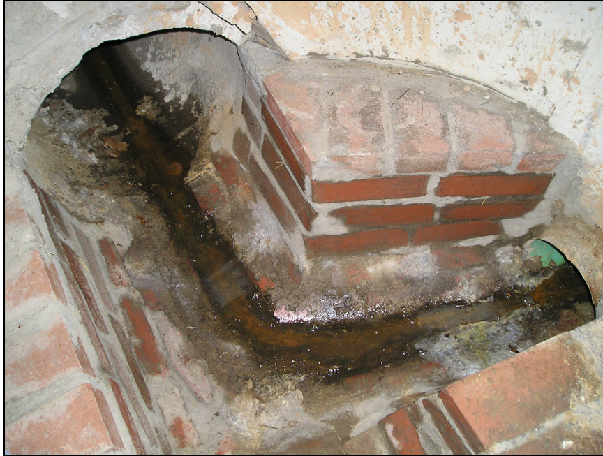
Figure 2-3. Manhole and flow splitter upstream of the Kenilworth cell. Flow enters from the 46 cm storm drain (top) and is directed to a 20 cm PVC pipe (right) that leads to the cell. During periods of extreme discharge, flow may bypass to the existing 46 cm pipe (bottom of image), which daylights to an existing ditch.
