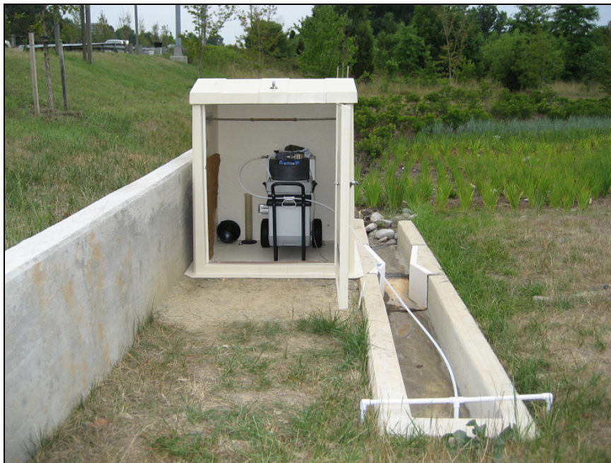
Figure 2-4. Inflow area for the Kenilworth Avenue cell, with sampler and housing, channel, and cutthroat flume. Samples are taken at the upstream end of the channel. Inflow level is measured at a prescribed point in the flume.
