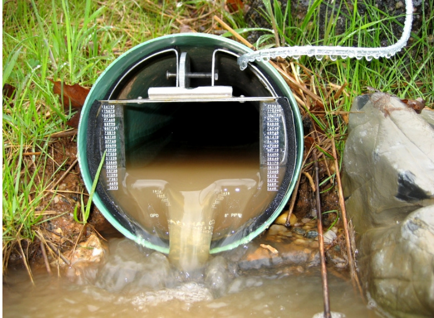
Figure 2-6. Outflow weir at Kenilworth cell (20 cm diameter). Outflow levels higher than the horizontal bar exceed the measurable range of the weir. Above this point, the level-to-flow rate conversion is undefined. Photo taken April 15, 2007.
