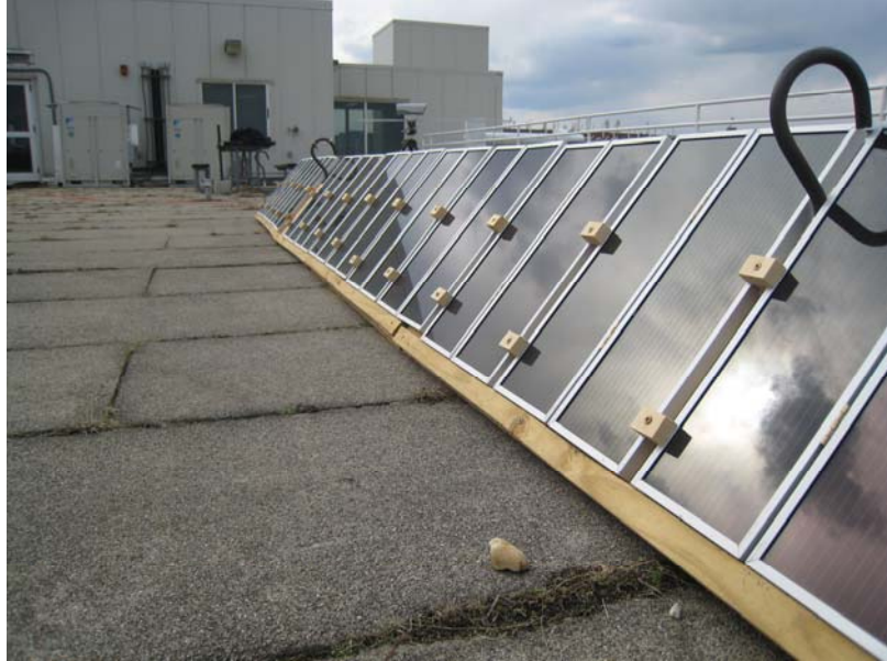
Figure 6: Panels mounted on the roof of the engineering building.
