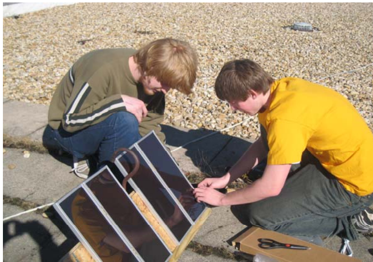
Figure 7: Team SHINE members fasten mounts to the hooks on the engineering roof.
