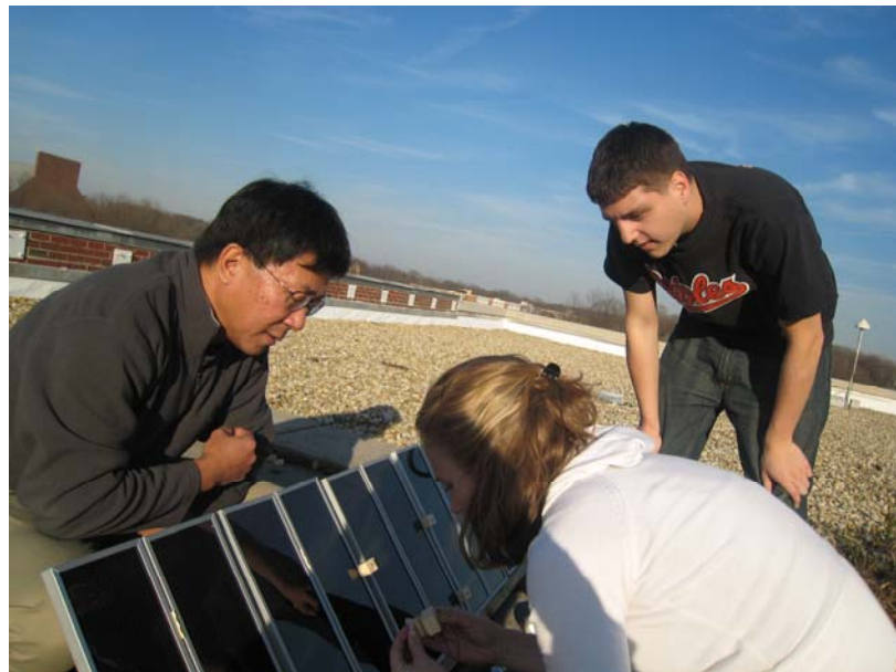
Figure 3: Team SHINE members mount solar panels on the roof of Martin Hall.
