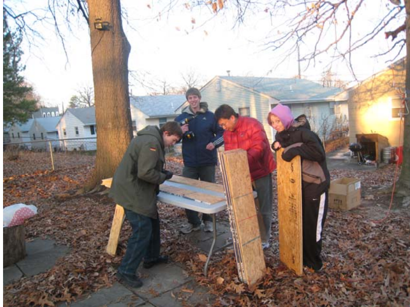
Figure 4: Team SHINE members build mounts for the panels.
