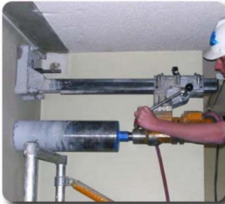
Figure 2-3: Drilling the Core
