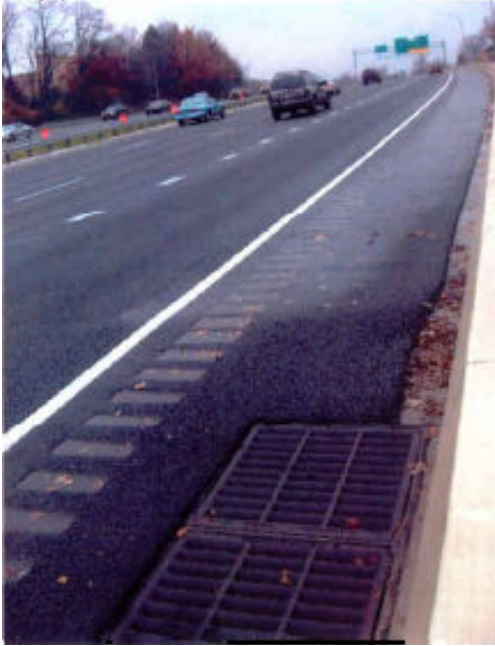
Figure 3-5. Inlet I-43 of BMP 3008 along I-83 NB
