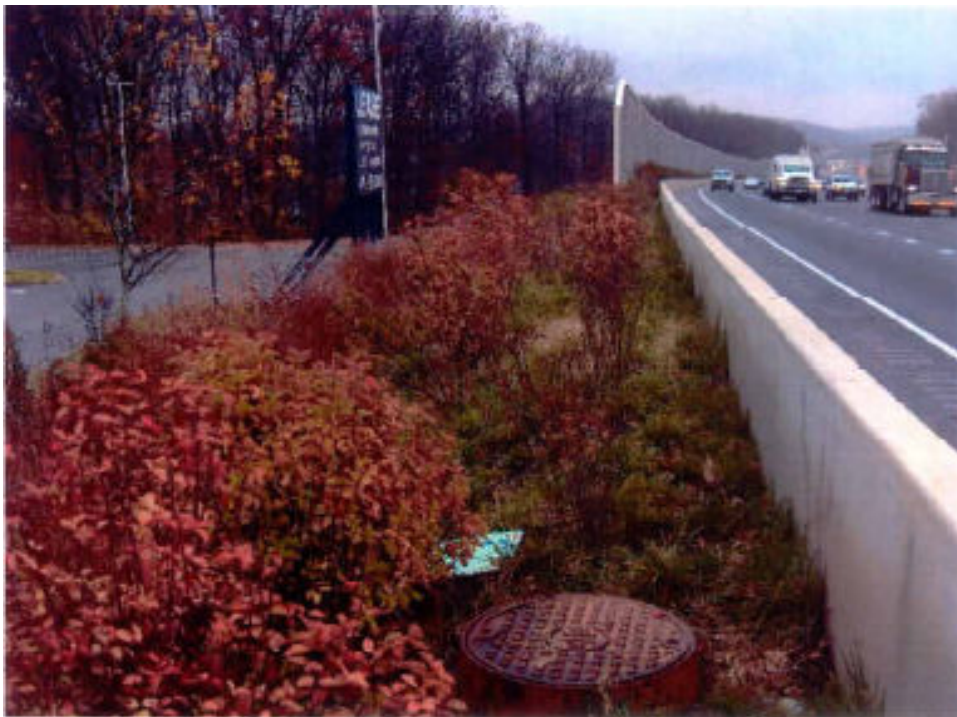
Figure 3-3. Study site BMP 3008 along I-83 NB
