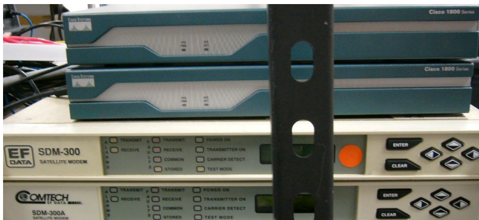
Figure 4-2. RF modem and routers
