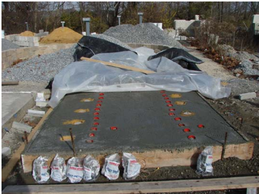
Figure 4.8 Slabs with cast-in-place cylinders, floating inserts and field cure cylinders Note: red marking are the pullout inserts; field-cured cylinders placed outside the slab; cast-in-place cylinders are within the slab.
