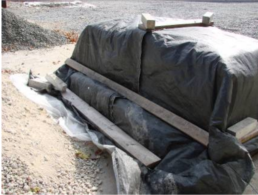
Figure 4.6 Concrete block curing in field.
